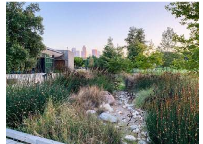
STORMWATER MANAGEMENT RAIN GARDEN
