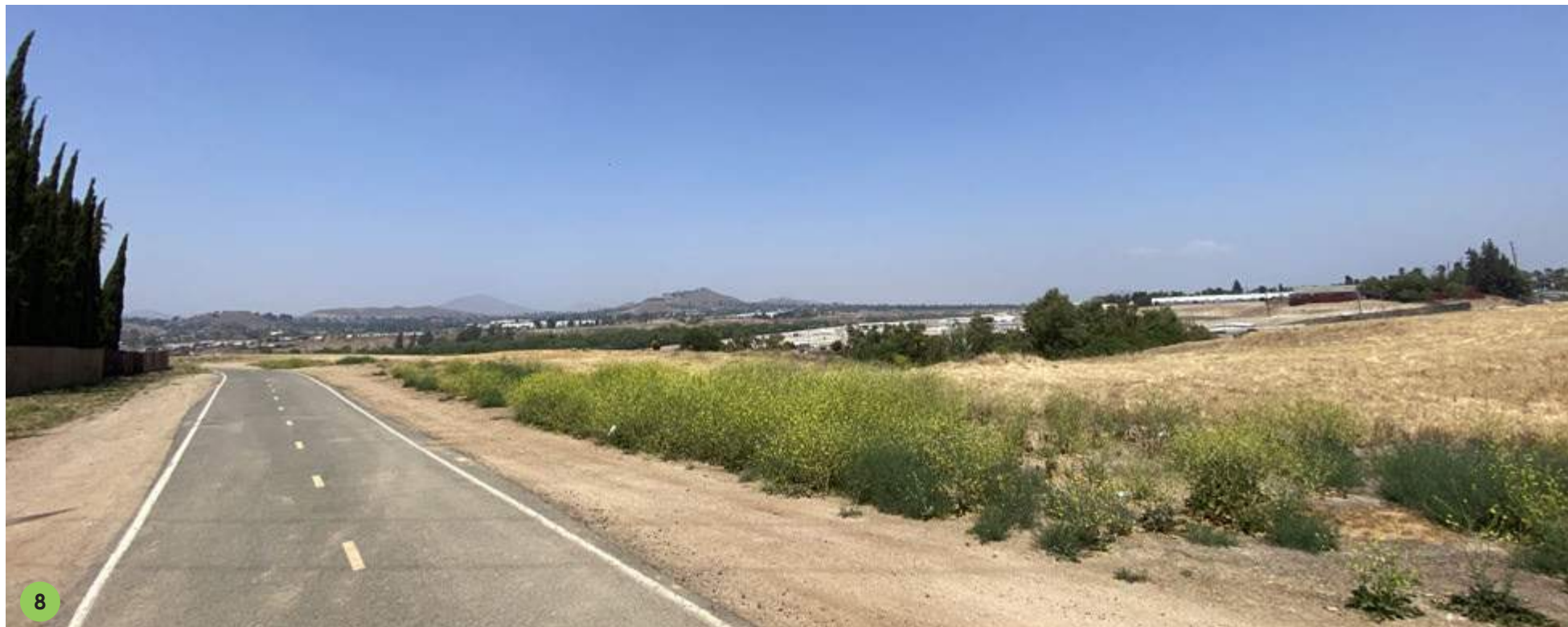
Existing Santa Ana River Trail
