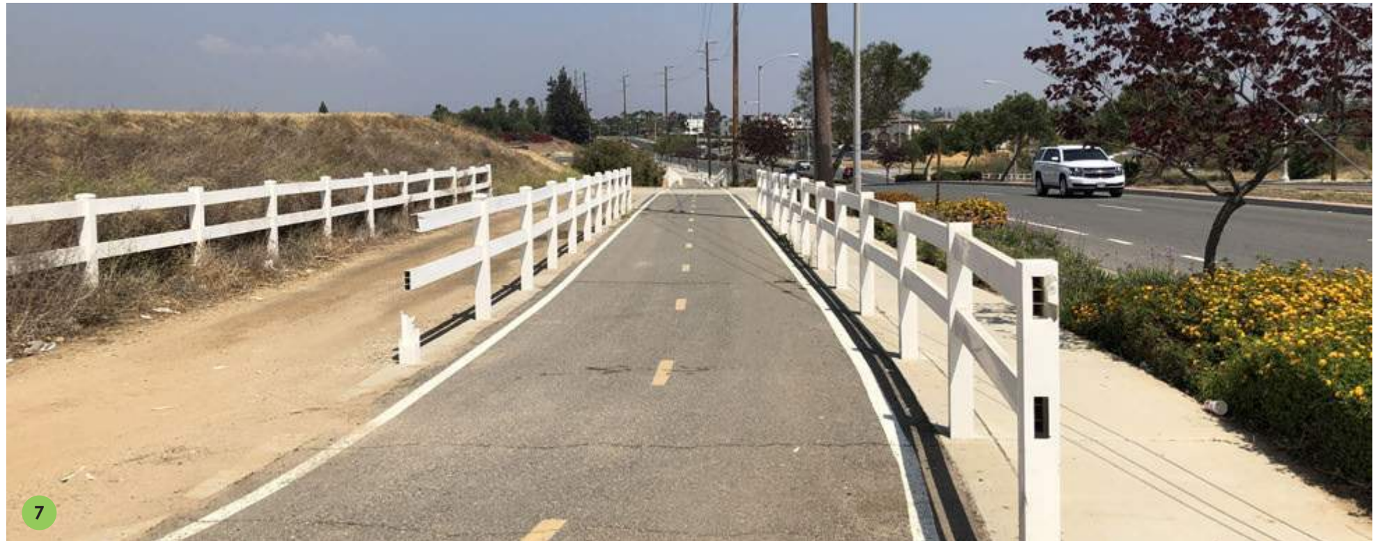
Existing Santa Ana River Trail and fencing along Jurupa Ave.
