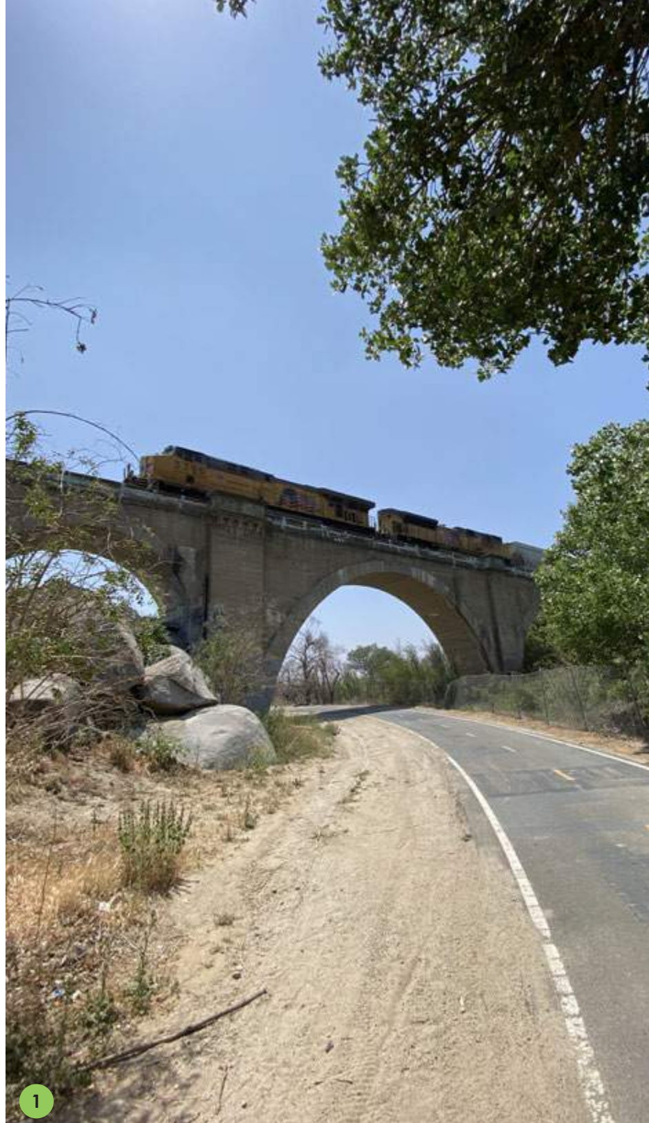
Existing Santa Ana River Trail under rail bridge
