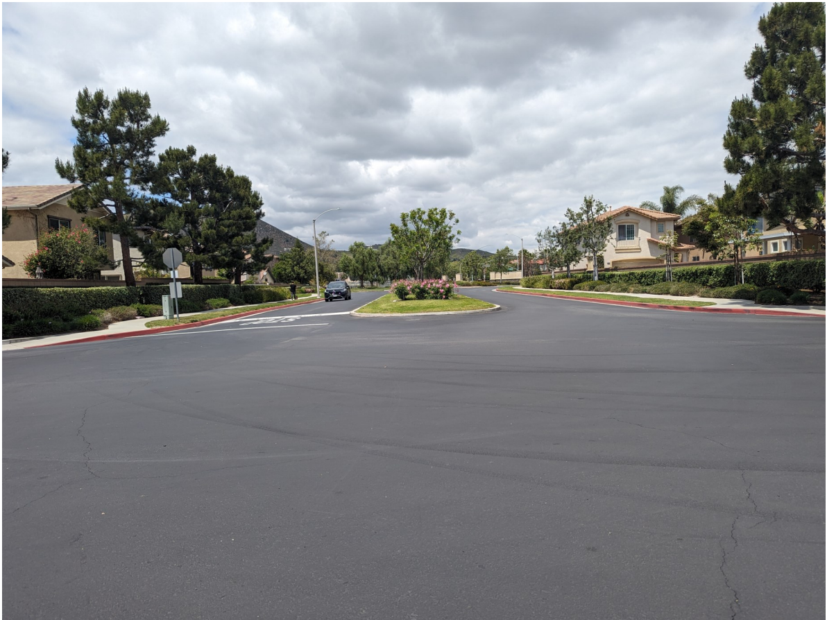
Westerly view of the Sierra Vista Avenue
