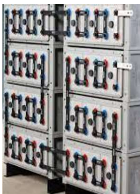
Typical Valve Regulated Battery Bank
