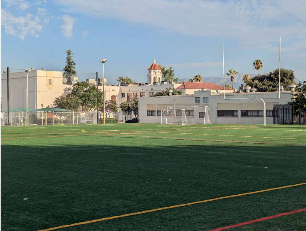
Figure 9 - Project site with historic structure in the distance; view from the Douglas Avenue looking northwest
