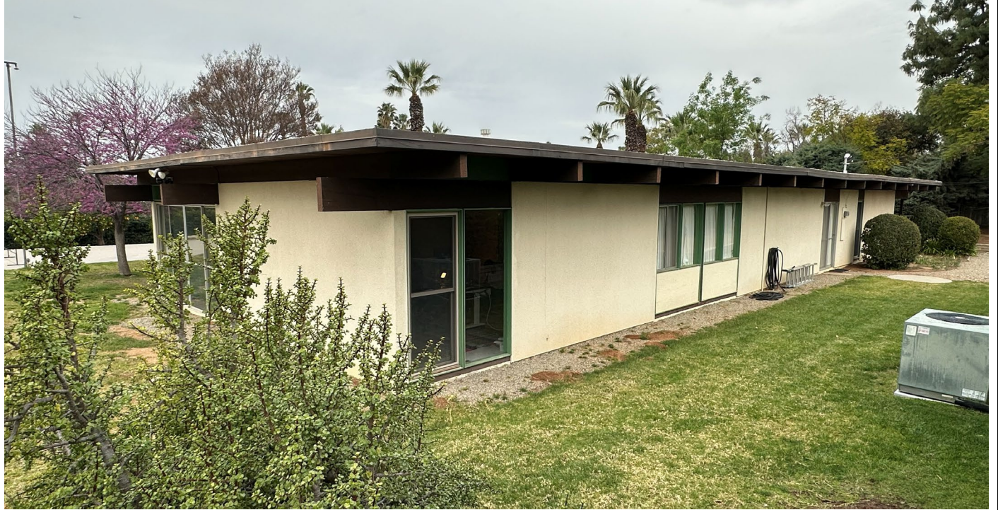
Rear and east side/rear elevation showing example of double-hung vinyl replacement of jalousie window in original opening, view northwest
