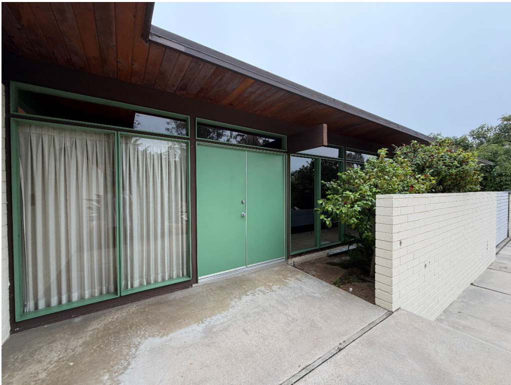
Figure 4 – Edie façade fenestration, eave, and roof beams behind freestanding garden wall, view southwest
