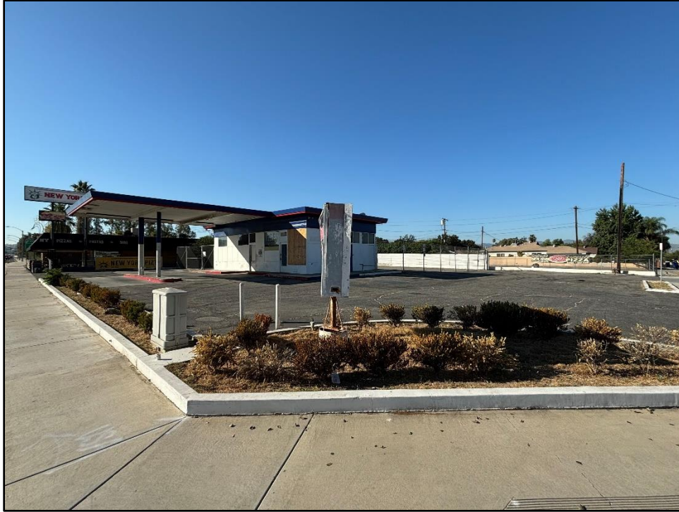
Looking southwest across the project site, from Van Buren Boulevard.
