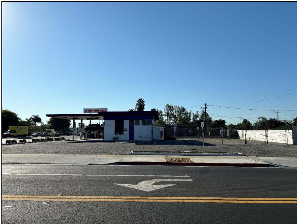
Looking south at the project site, from Primrose Drive.
