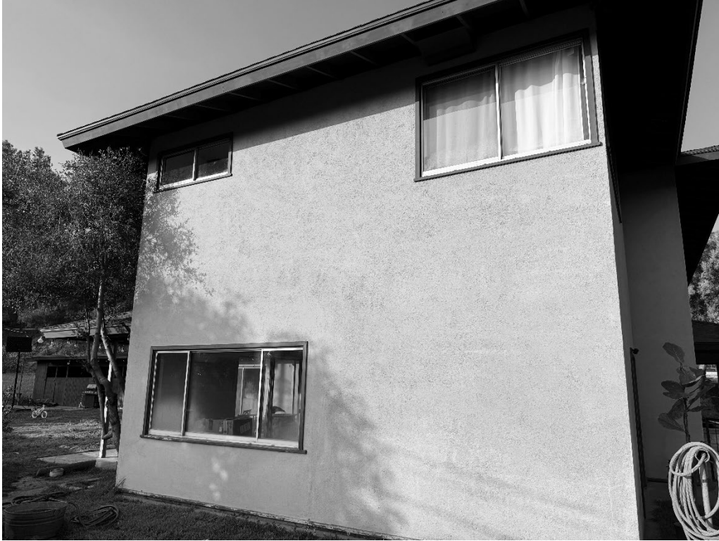
Figure 15 - East elevation, 1973 two-story addition
