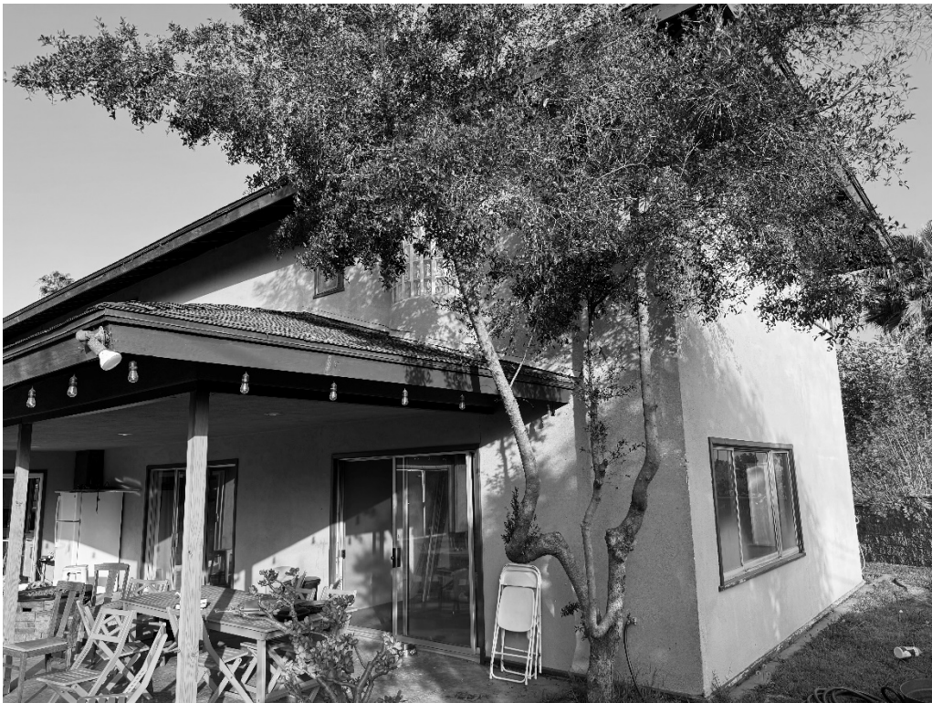
Figure 14 - South and east elevation, with 1973 two-story addition
