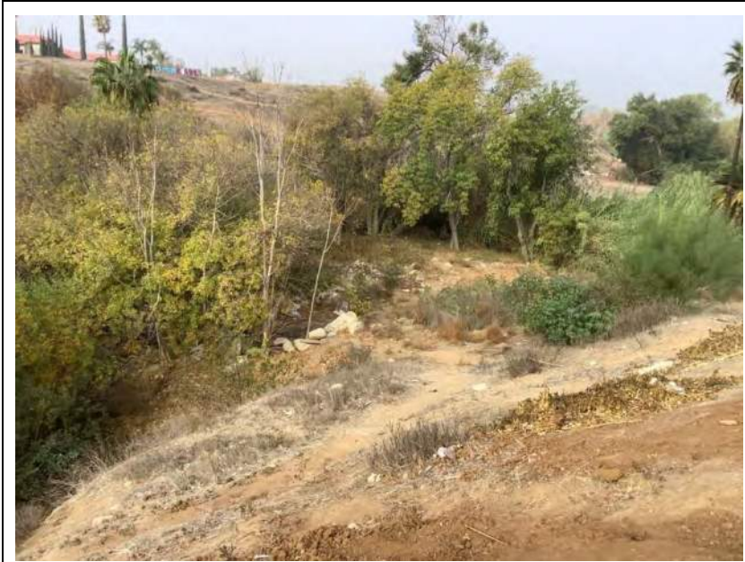
Photograph: 19 Photo Date: 12/3/21 Location: Feature 3 – Hole Creek, Jurupa Ave. Trailhead Direction: Northwest Comment: Looking downstream at the east side of Feature 3.
