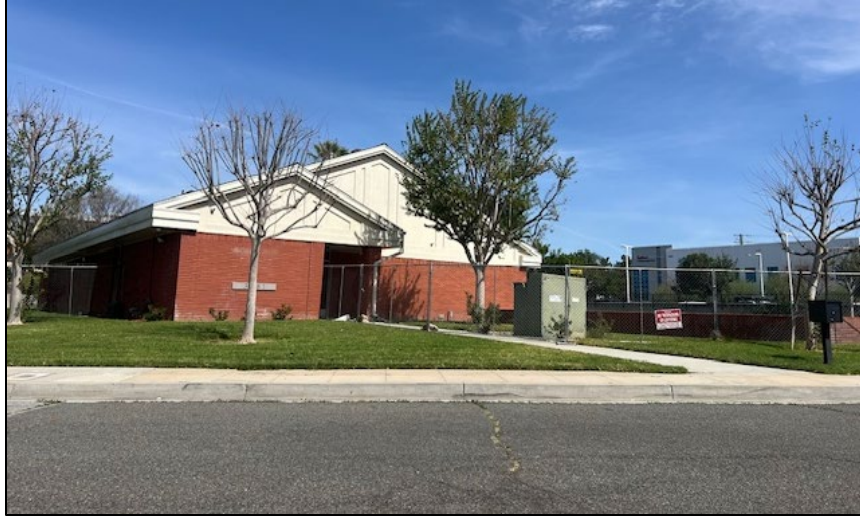
Looking northeast at the project site; from Prospect Avenue
