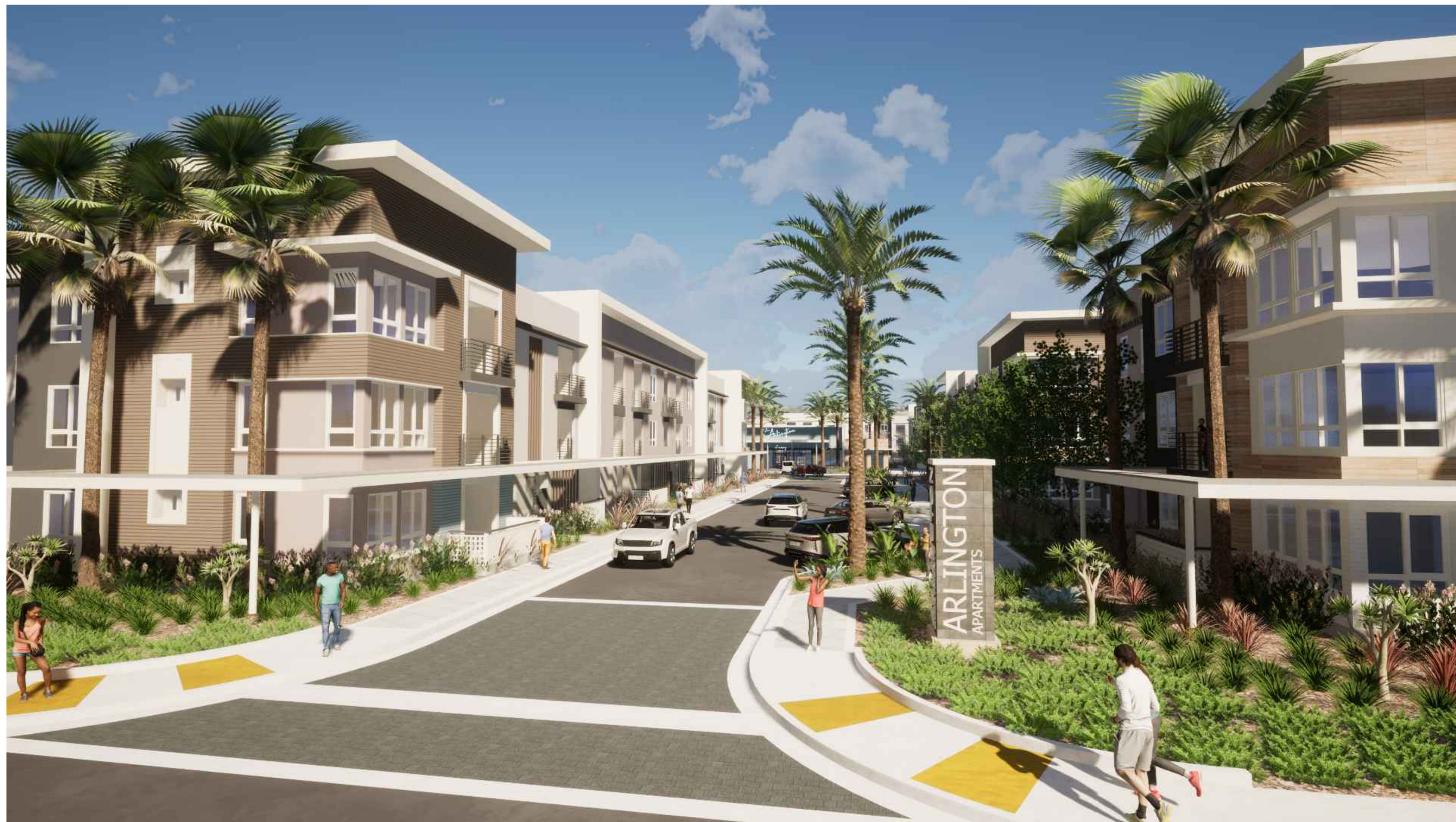
MAIN ENTRY | STREETER AVENUE
