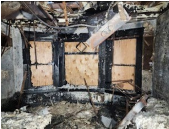
Photo 9. One of the bay windows (2024).
