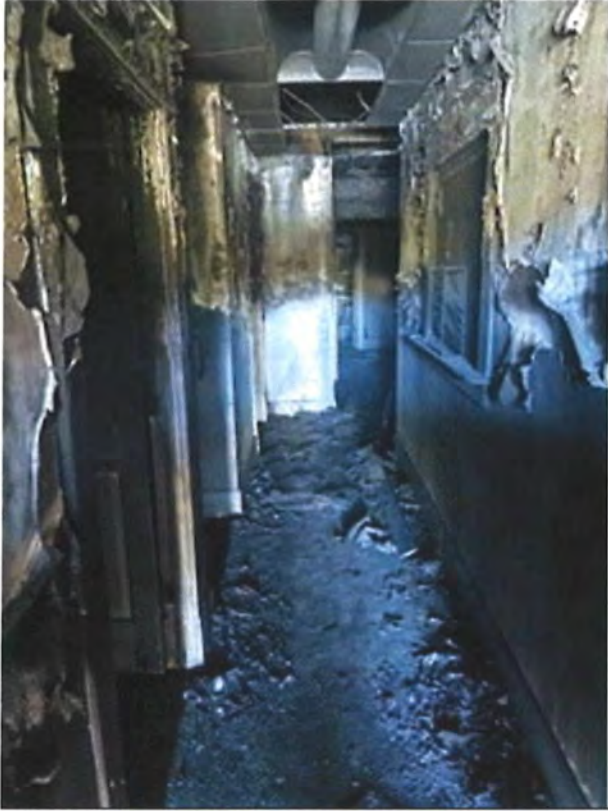
Photo 7. Entry hall taken from front door (2024).
