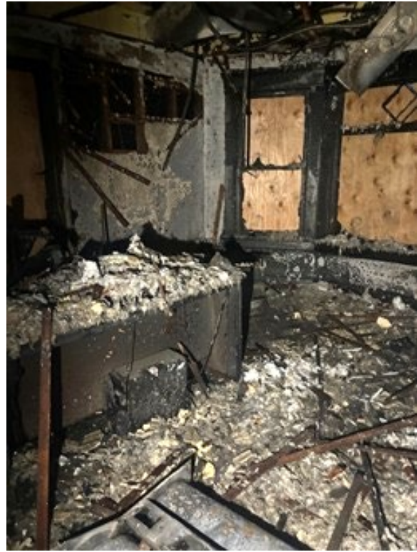
Photo 8. Office with bay window (2024).
