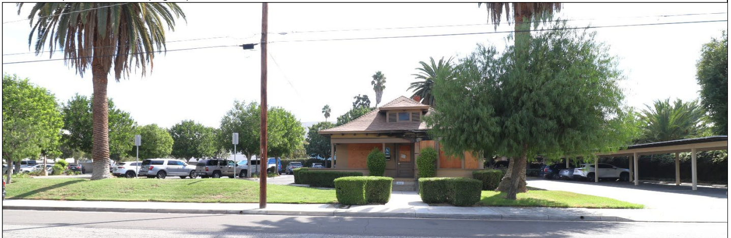
Overview of setting showing the extended lawn area, parking lots, wide driveway, carport, and trees. View east (10/7/24).
