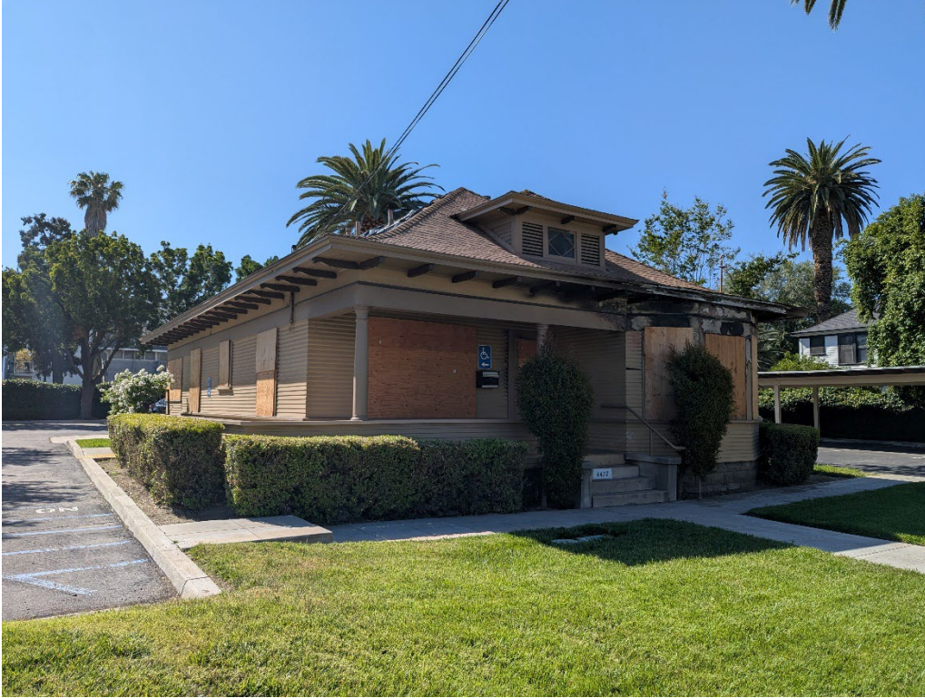
Figure 1 - Front facade, view looking southeast
