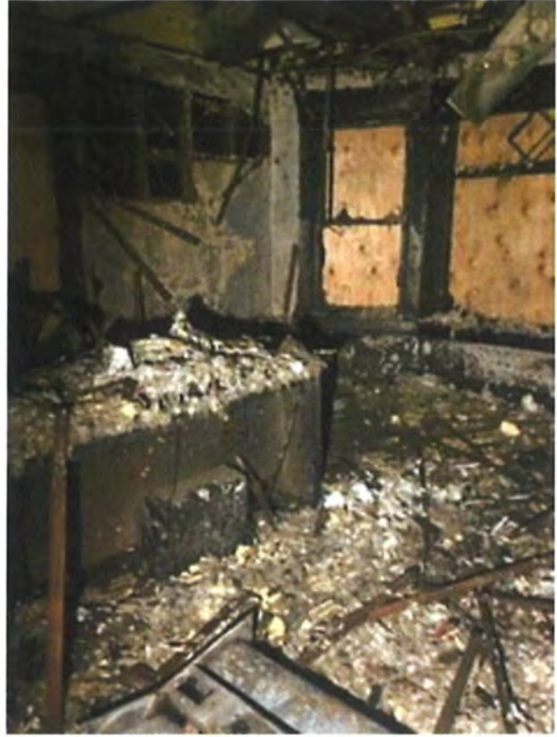
Photo 8. Office with bay window (2024).
