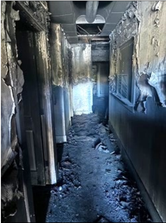
Photo 7. Entry hall taken from front door (2024).
