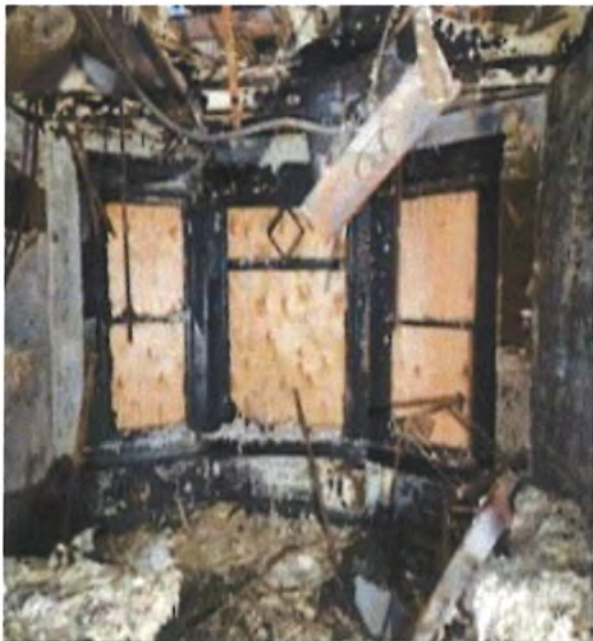
Photo 9. One of the bay windows (2024).
