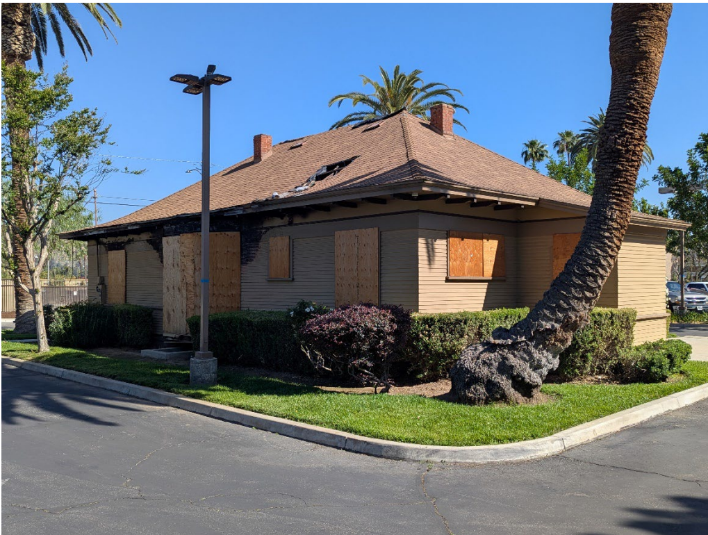
Figure 4 - South and east elevations, view looking northwest
