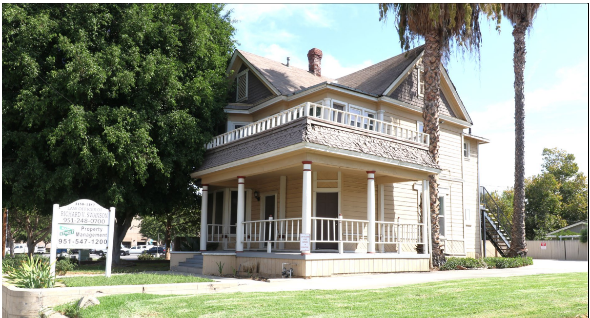
Photo 13. Offices at 4480–4482 Main Street, view northeast (10/7/24).
