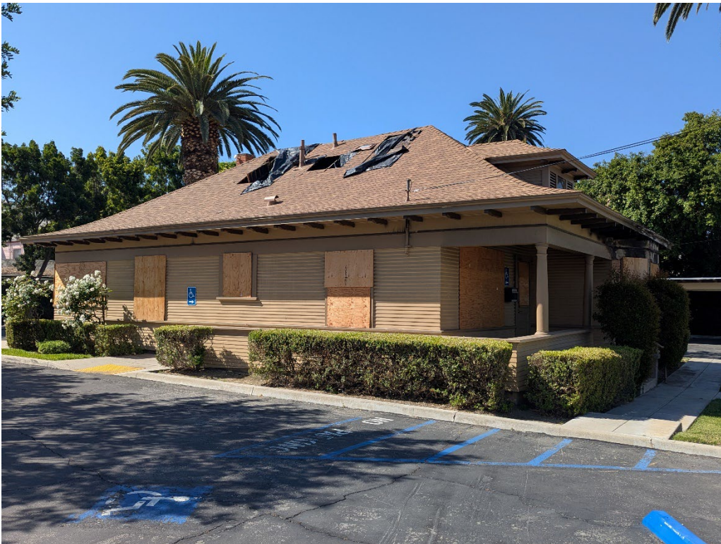
Figure 6 - North elevation, view looking south
