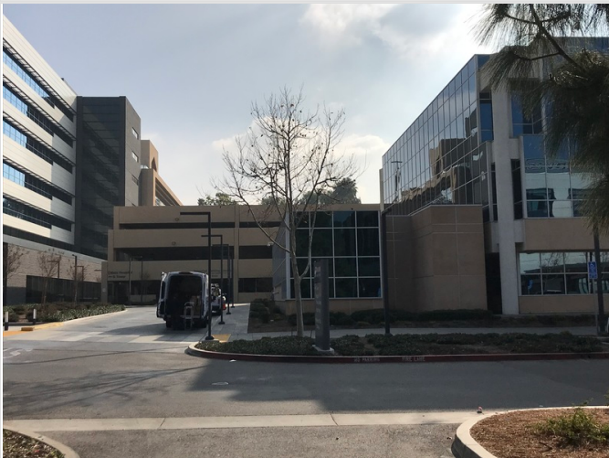
33. East adjoining property
