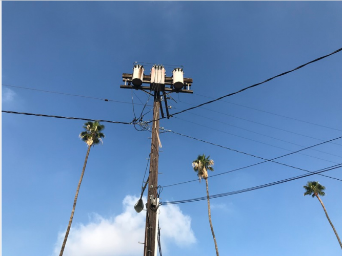
31. Pole-mounted transformers
