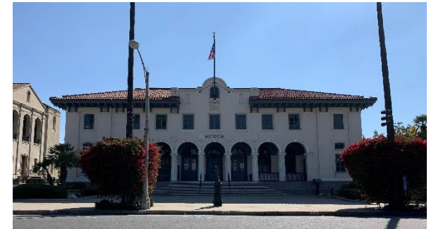
Maintaining 4 historic sites (7 sites total)
