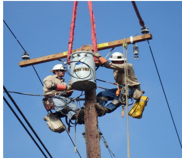
Transformer and Cross-arm Replacement
