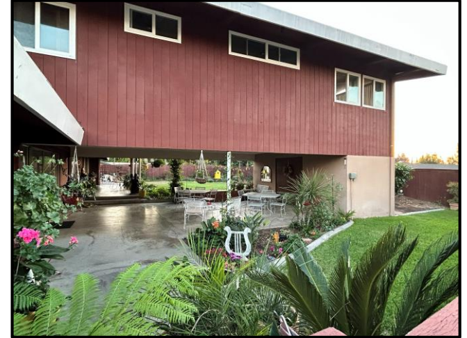
Second Story with under patio
