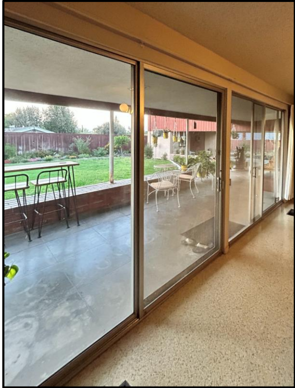
Original Aluminum Sliding Doors, example of original window material
