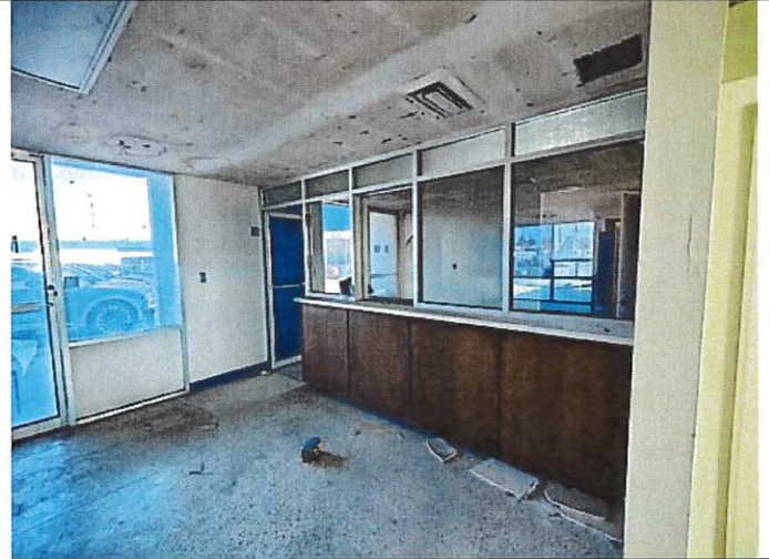
Rear of building (northwest area), office space.
