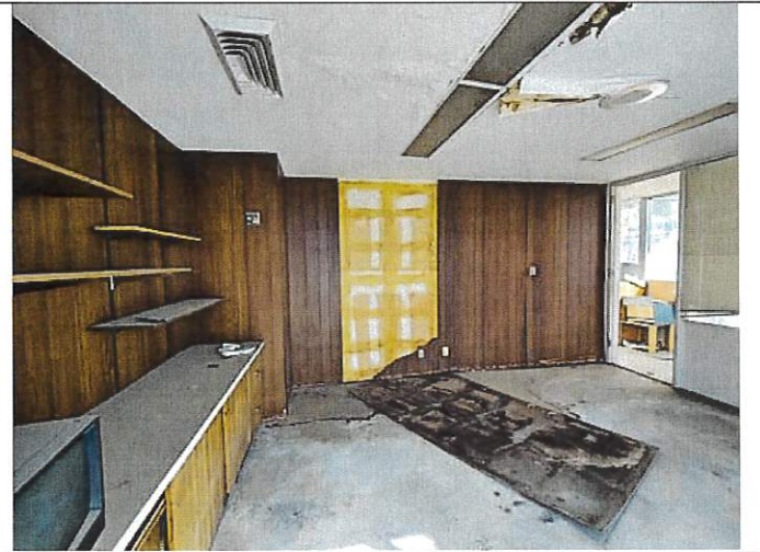
Rear of building (northwest area), office space.
