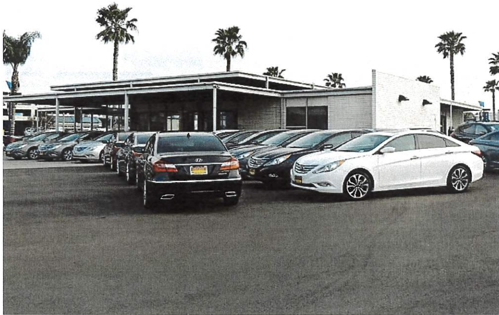
View looking South (March 2013)
