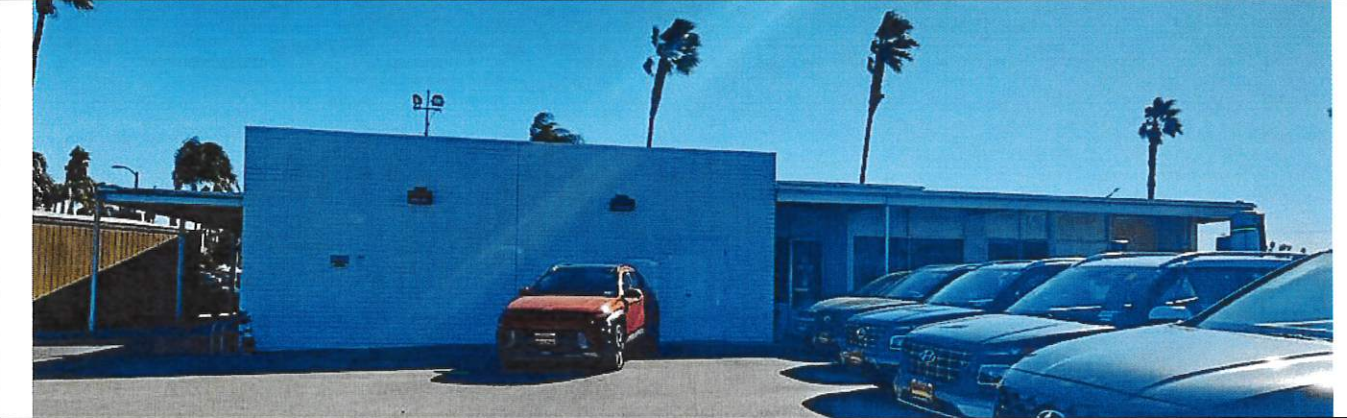
Northwest elevation, facing southeast.
