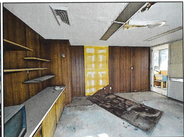
Figure 7. Rear of building (northwest area), office space.
