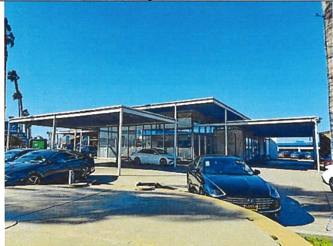
Oblique southeast corner, facing northwest.
