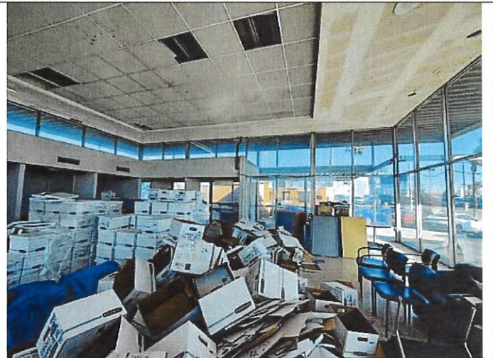
Main lobby/showroom interior, facing north.
