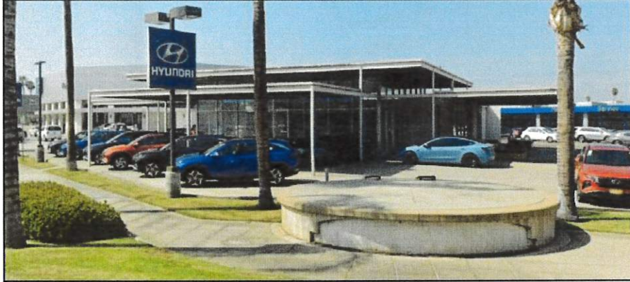
Figure 4. 2022 Street view of the showroom to be demolished as part of Project Source: Google Maps
