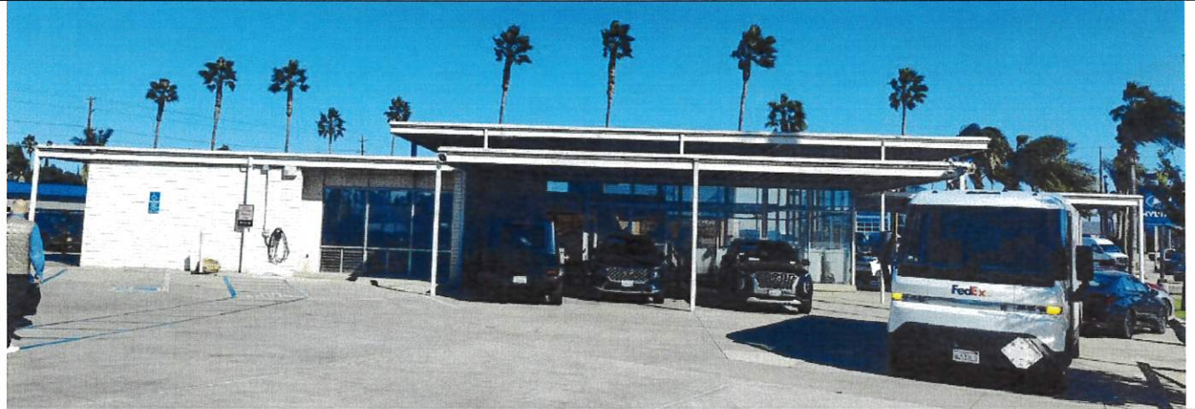
Southern elevation, facing northeast.
