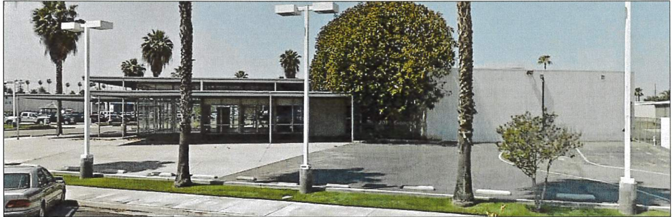
Northeast elevation. Original building configuration prior to demolition of the southern block of the building in 2012.
