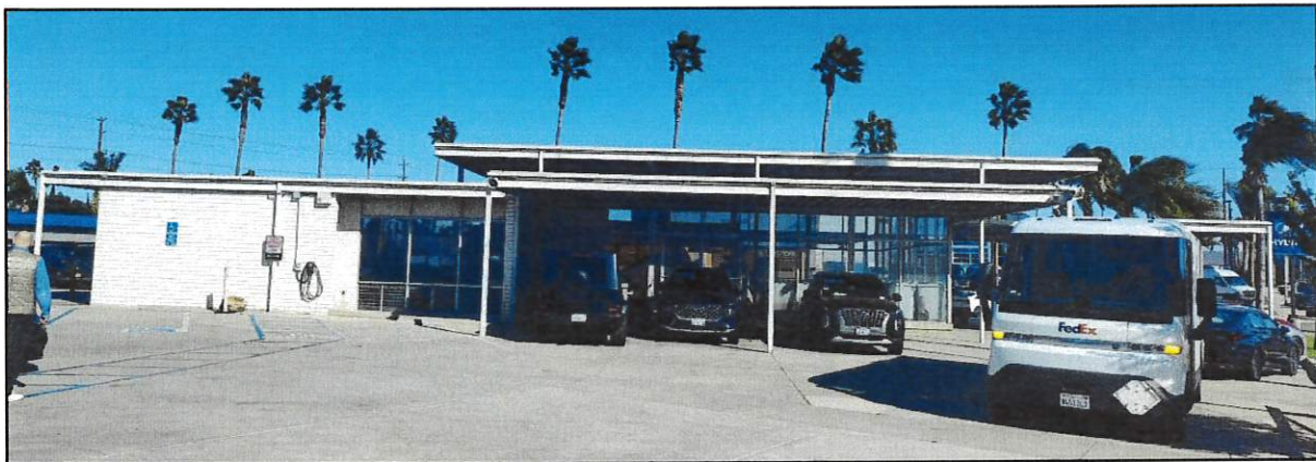
Figure 9. Southern elevation, facing northeast.
