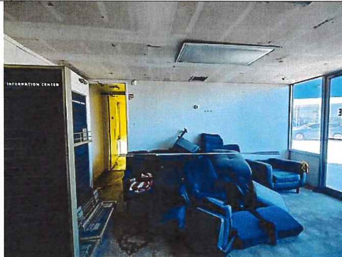
Rear of building (northwest area), office space.
