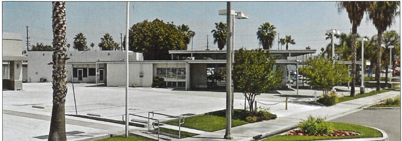
Southwest elevation. Original building configuration prior to demolition of the southern block of the building in 2012.
