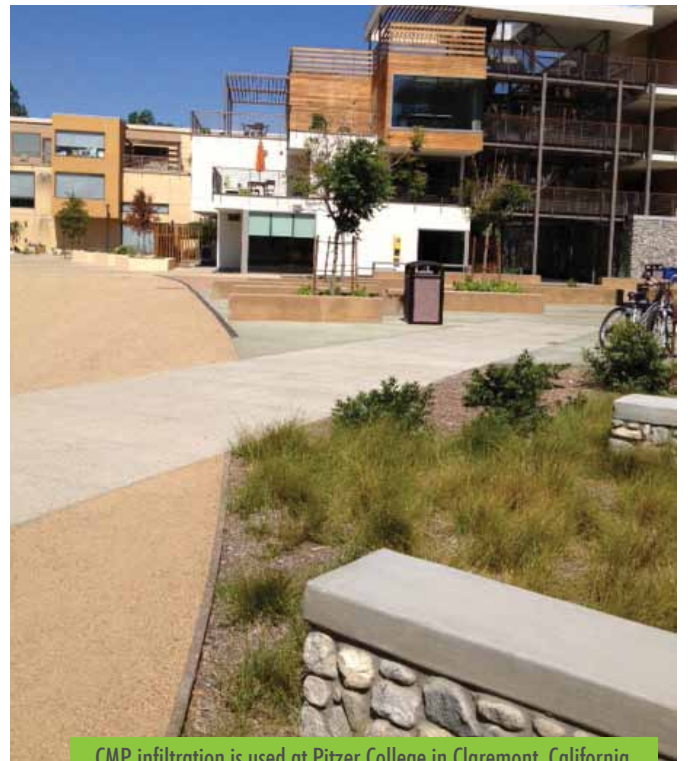
CMP infiltration is used at Pitzer College in Claremont, California.
