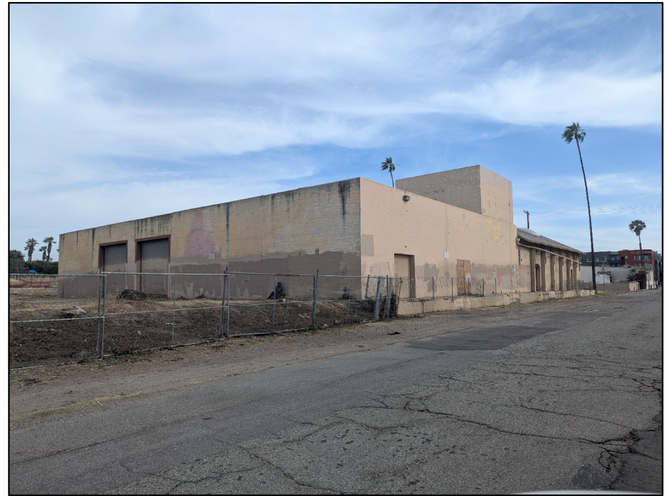
Non-original addition, looking southeast
