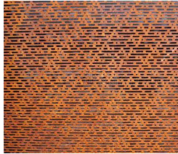
PERFORATED STEEL HUES OF RUSTED RED & BROWN OCCURS AT STAIR TOWERS - ALL LEVELS
