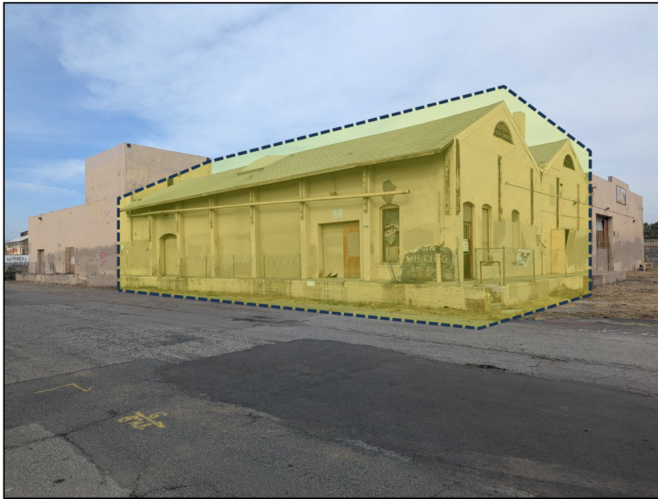
West and South Elevation, looking northeast
