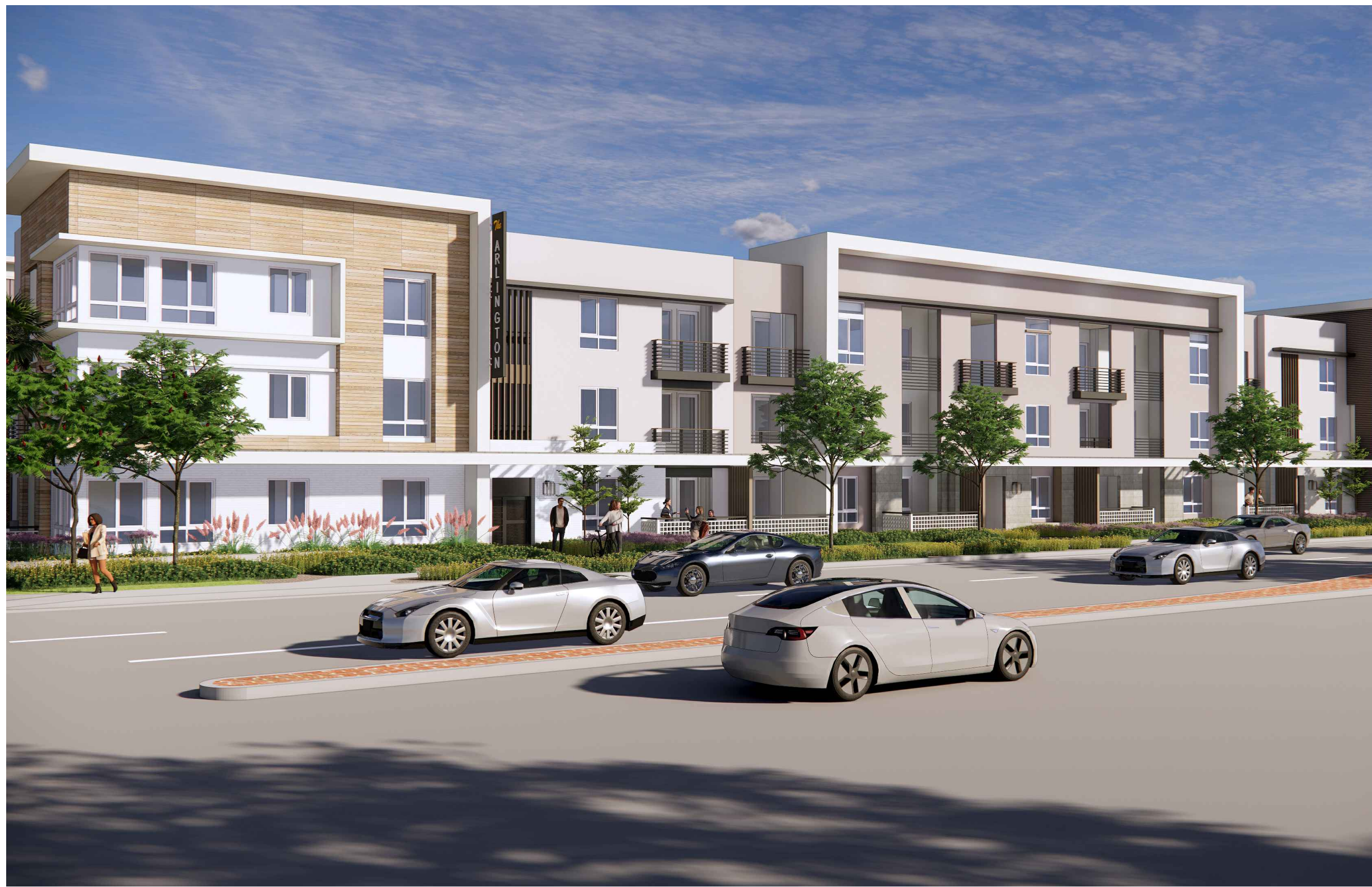
VIEW OF BUILDING 9 ALONG STREETER AVE. 1
