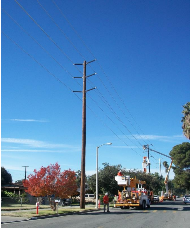
69kV overhead sub-transmission line work
