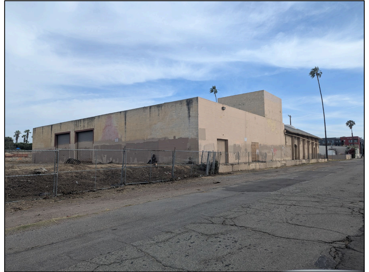
Non-original addition, looking southeast
