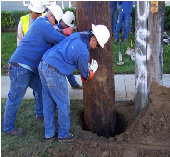
Typical pole and transformer replacement by RPU crews
