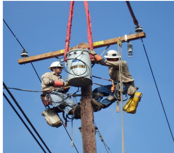
Typical pole and transformer replacement by RPU crews
