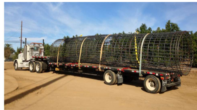
REBAR CAGE READY TO BE OFFLOADED AT JOB SITE
