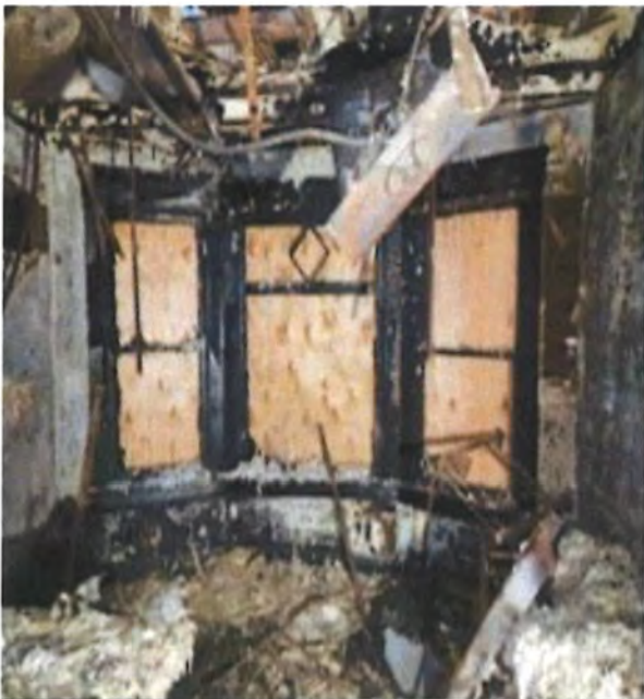
Photo 9. One of the bay windows (2024).
