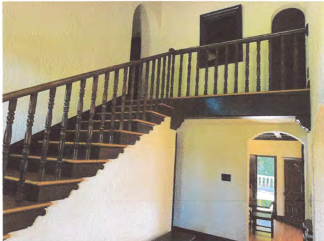
Interior rotunda stair, balcony, doorways, view NE
