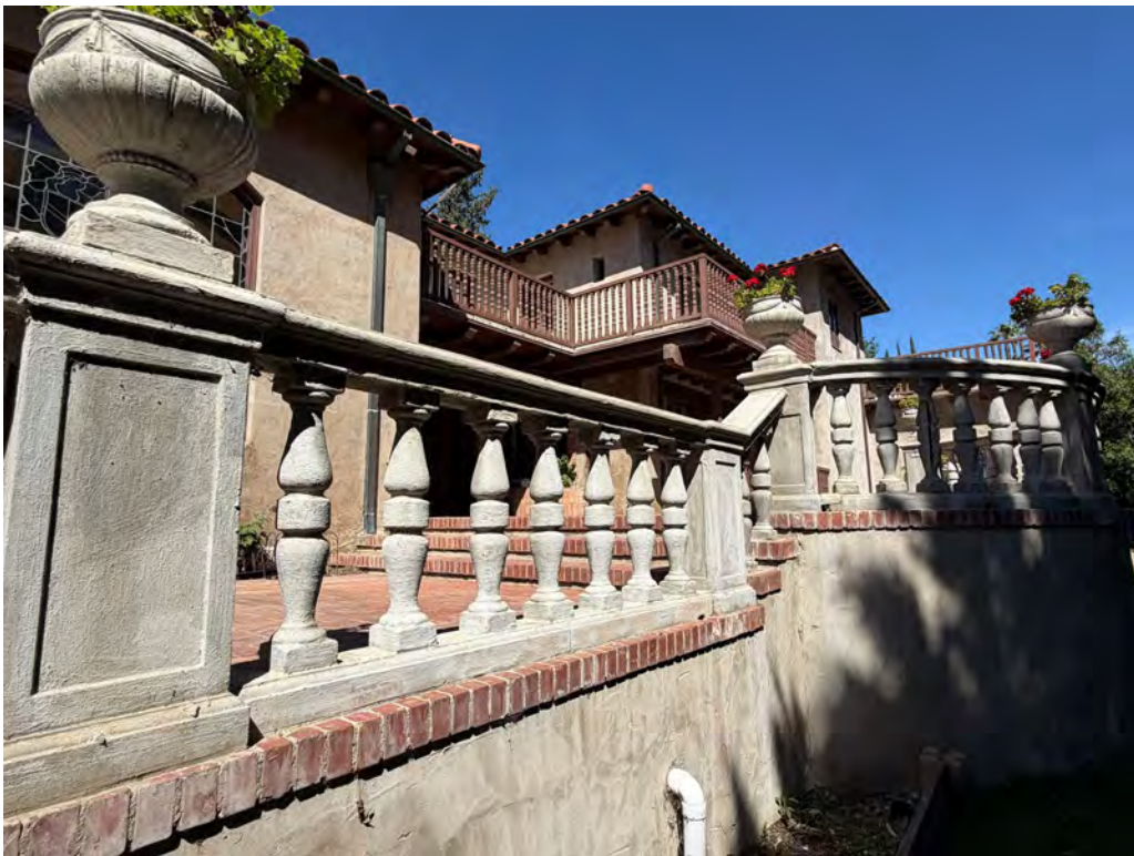
Figure 4 - Rear patio balustrade, view looking north
