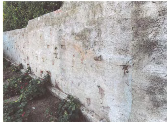
Front perimeter wall detail (1890s-1904), view SW
