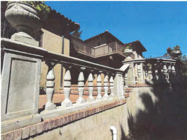
Rear elevation and patio detail, view N/NW
