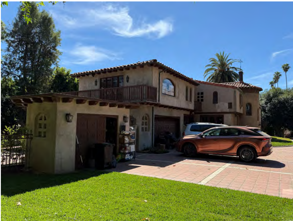
Figure 2 - West elevation, view looking southeast
