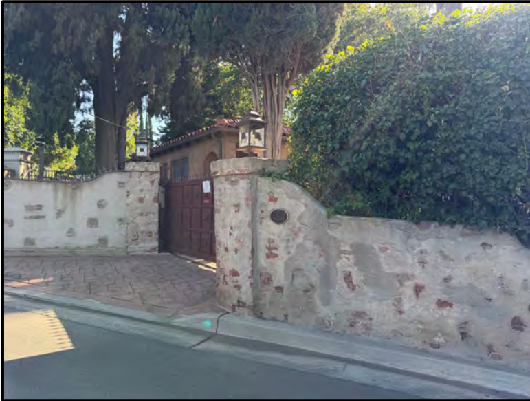
Perimeter wall and gate house
