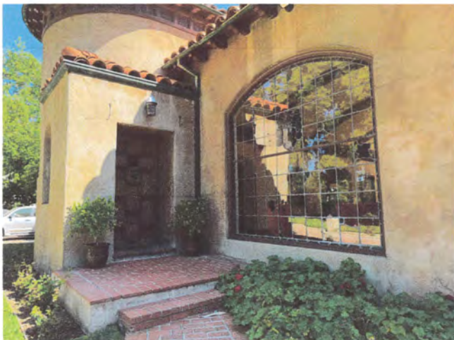
Entry and fenestration detail, view N/NE
