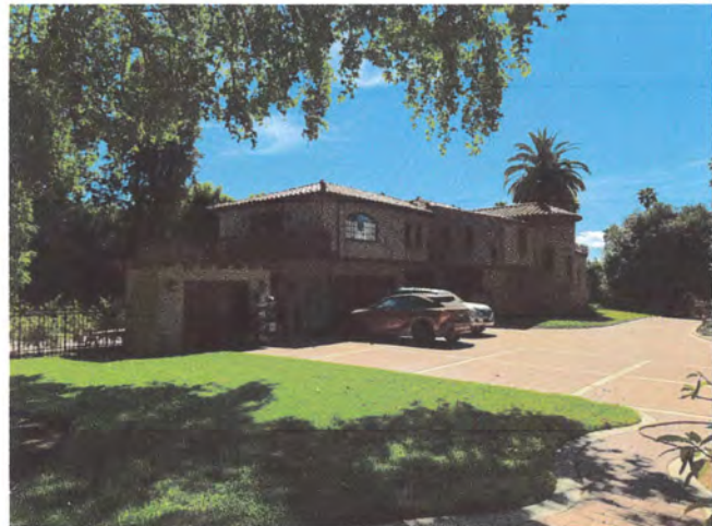
Northerly side elevation and façade, view SE
