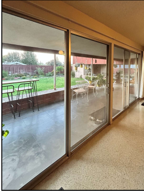
Original Aluminum Sliding Doors, example of original window material
