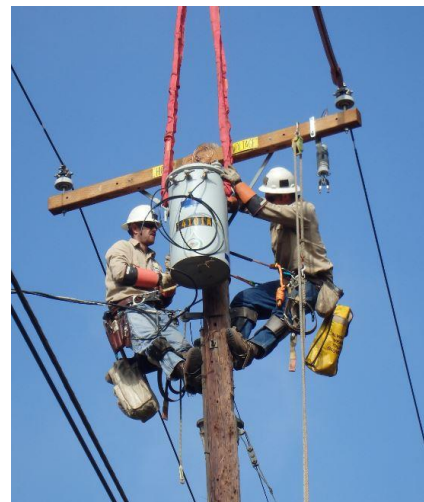
4-12kV Conversion – Transformer and Cross-arm Replacement
