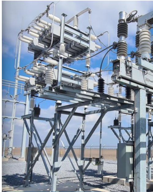
Typical 66 kV Capacitor Banks
