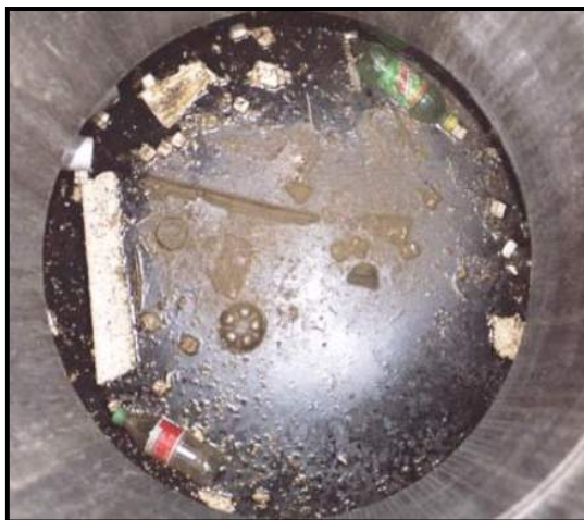
Floatable debris in the Aqua-Swirl®
