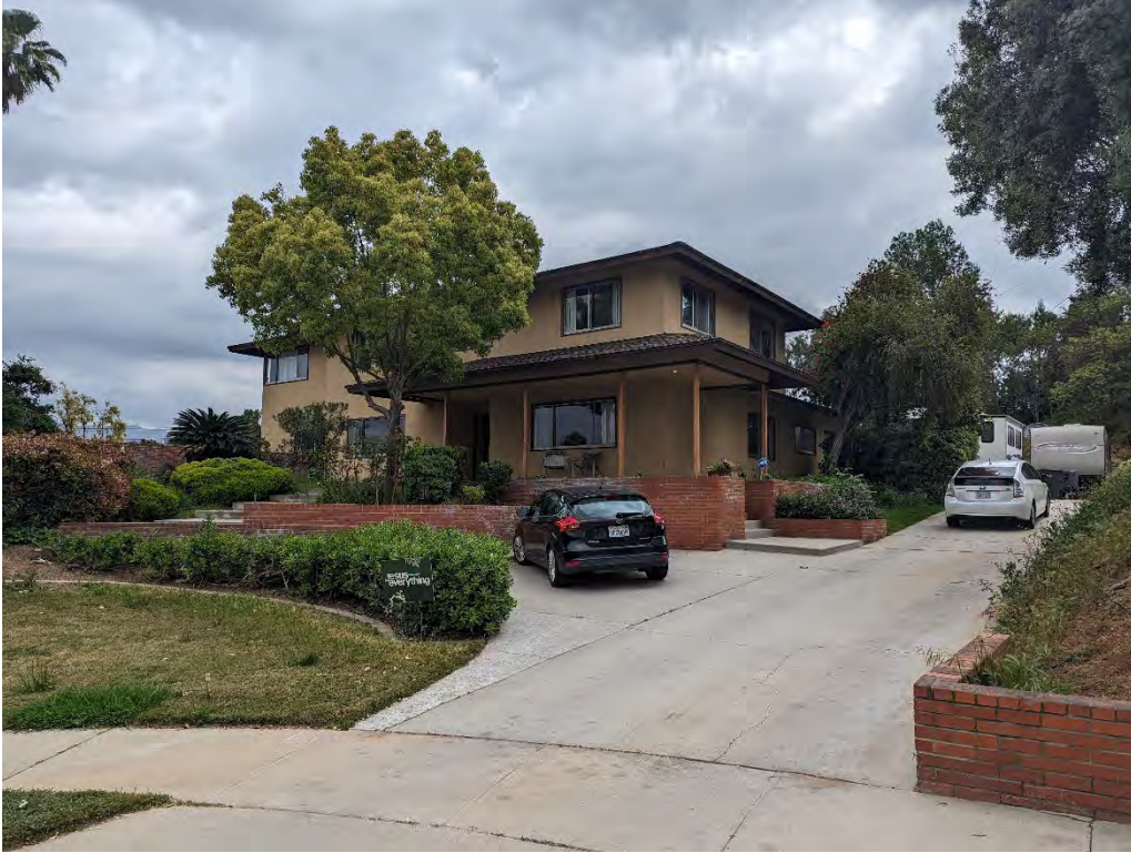
Figure 1 - North (front) elevation, view from street
