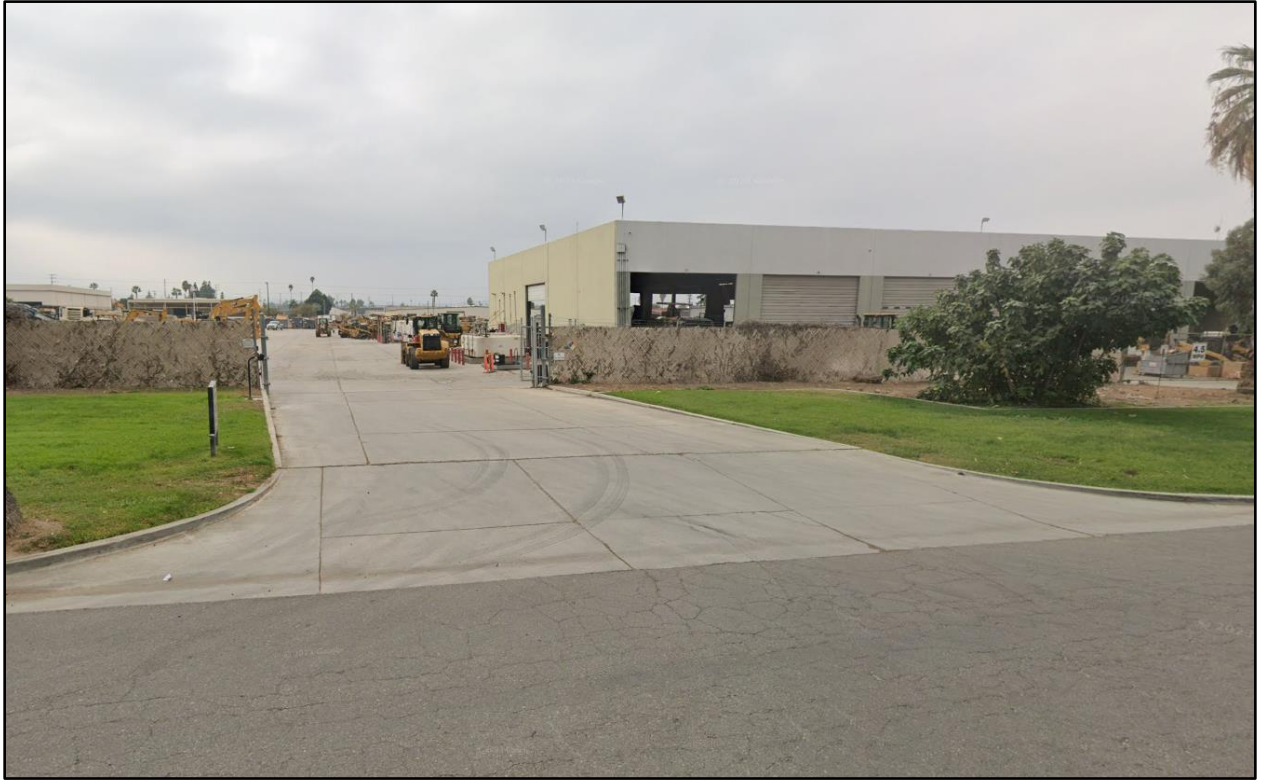
View of northerly entrance along Citrus Street
