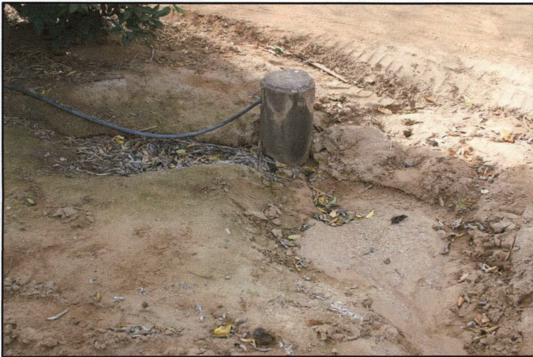
Example of low-profile standpipe irrigation head; these are placed along South-eastern (upslope) edge of the orchard and across the middle (Close-up)
