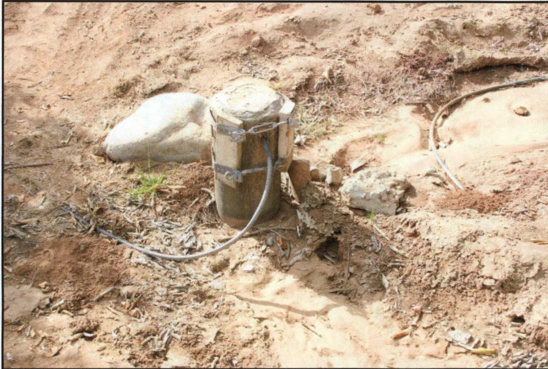
Another example of standpipe irrigation head (Close-up)
