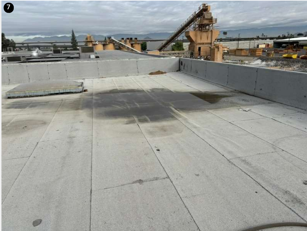
7 Additional ponding near perimeter, not near a drain channel.
