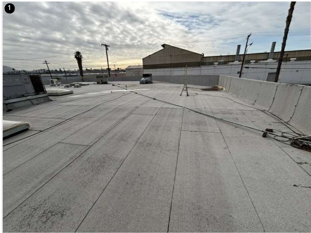
Overview of 2880 Hulen PI Built up roof on wood deck.
