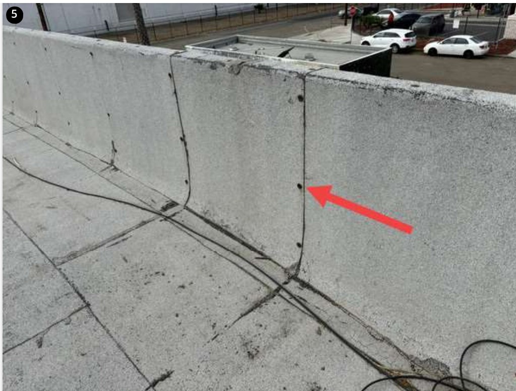
Parapet cap sheet mechanically fastened, fasteners fully exposed.
