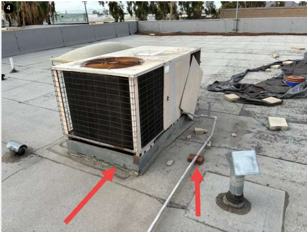
Improper flashing around HVAC unit and drains on wood blocks.
