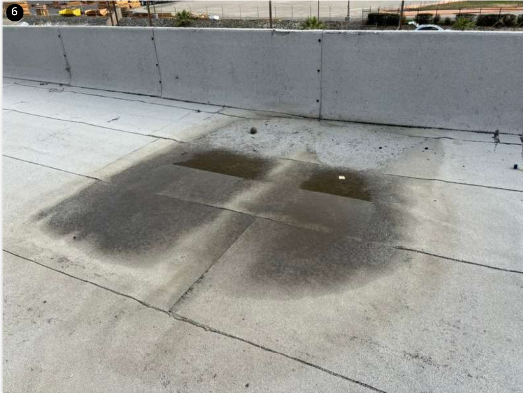
6 Ponding and mineral loss in middle portion of roof near perimeter. This location is not near a drain, roof slope to be reviewed.
