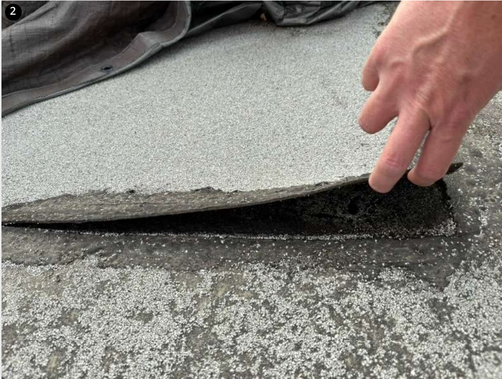
Open seams on cap sheet, allowing water to flow freely under waterproofing membrane.
