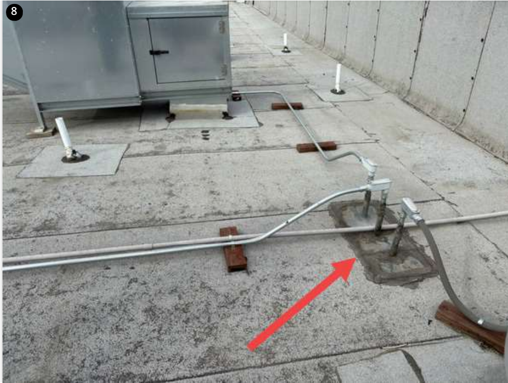
Penetrations not properly flashed in.
