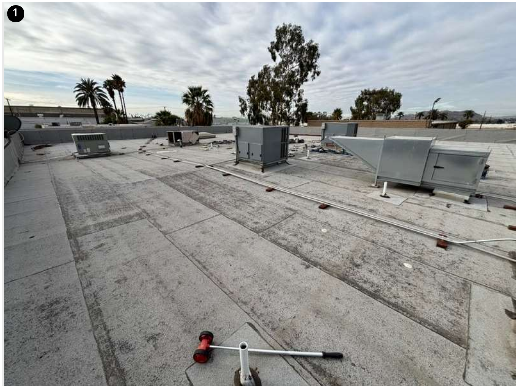
Overview of 2801 Hulen Pl Built up roof on wood deck.
