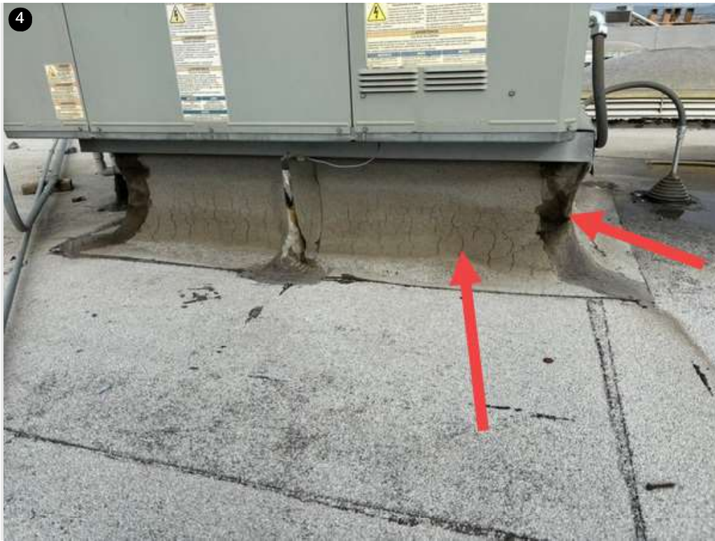
Adequate curb height, cap sheet wearing and mastic failing.
