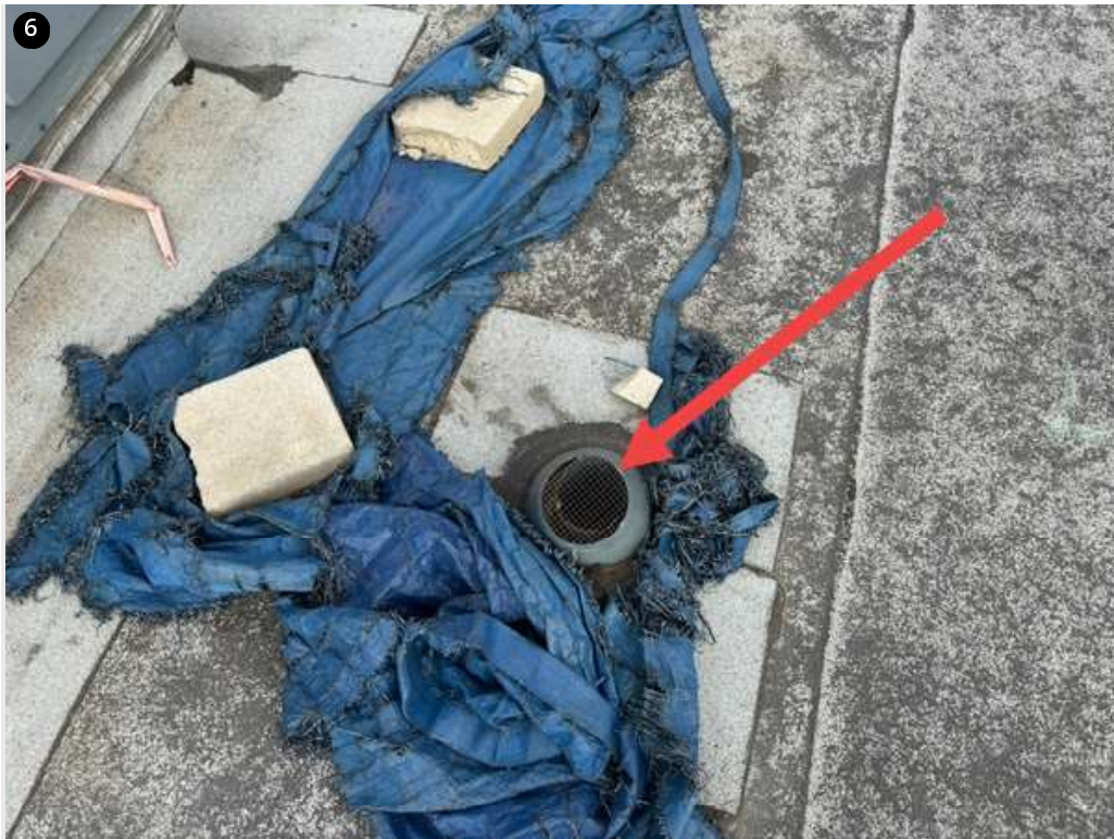
Multiple exposed vents.
