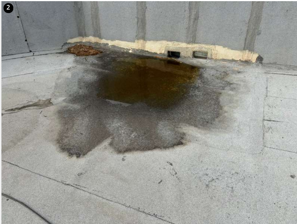
Ponding near southwest drain. Deck feels soft and possibly compromised in ponding areas.
