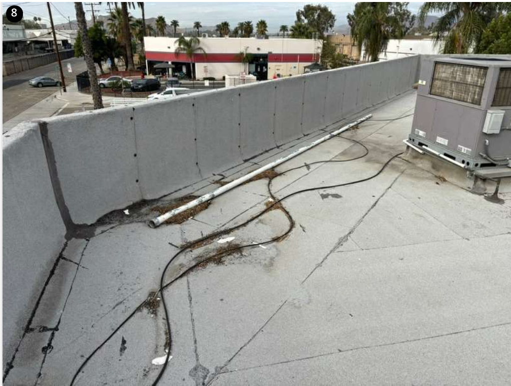
Conduit and debris lying on roof field.
