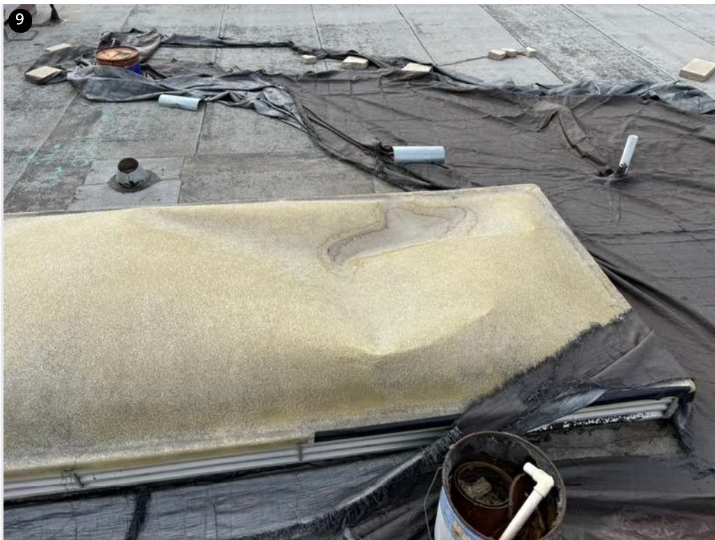
Damage to skylight.
