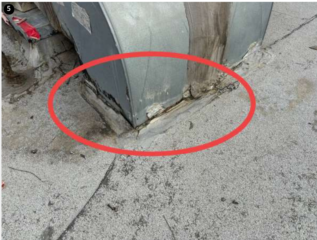
Failing mastic around exhaust.
