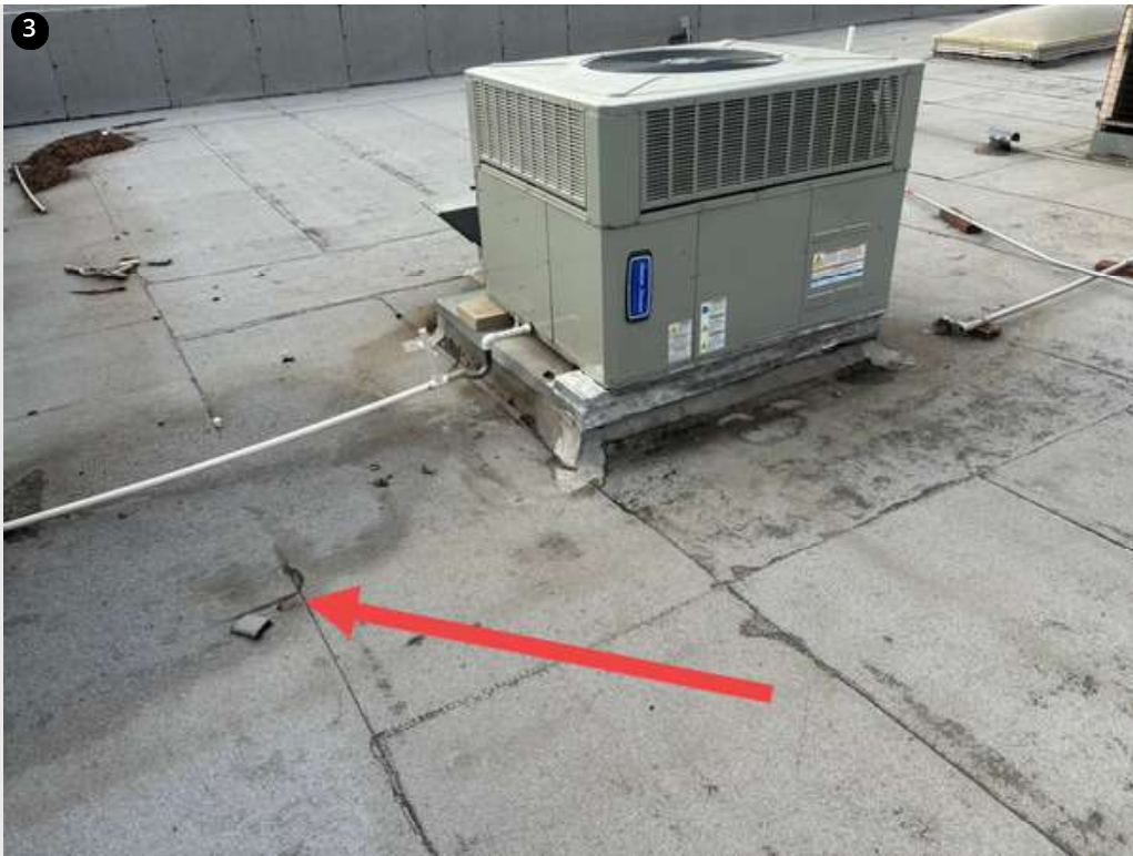
Significant mineral loss in drain channel.
