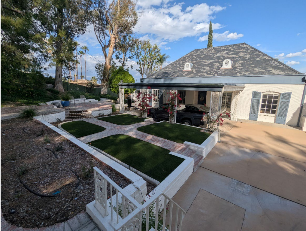
Figure 1 – Main façade (west) Elevation, view looking northeast
