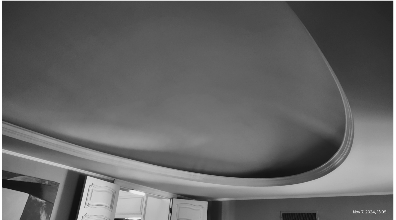
Figure 9 - Entry interior - oval recessed ceiling
