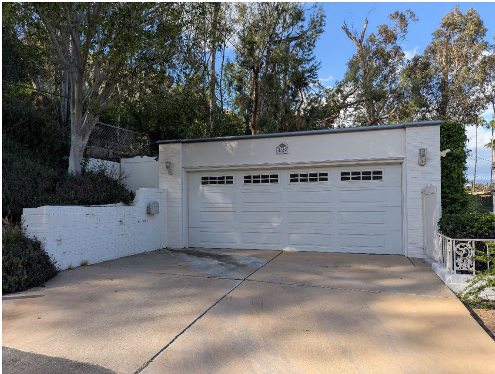
Figure 10 - Detached two-car garage
