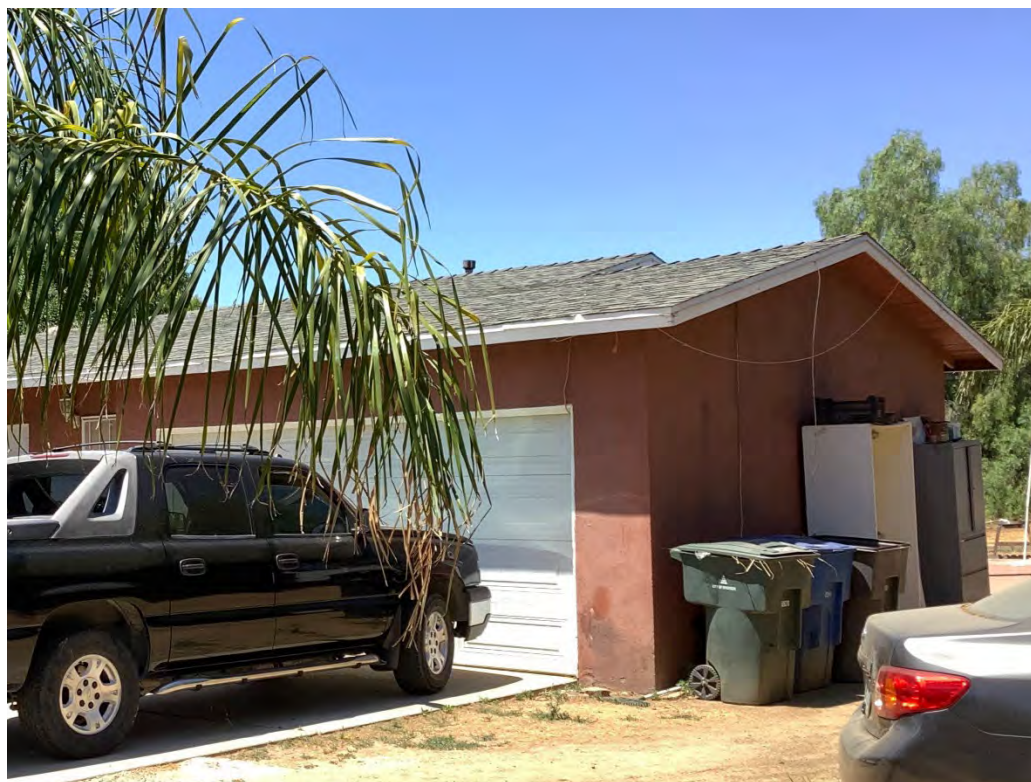
Figure 15. View of 4618 Jones Avenue, looking toward northwest.
