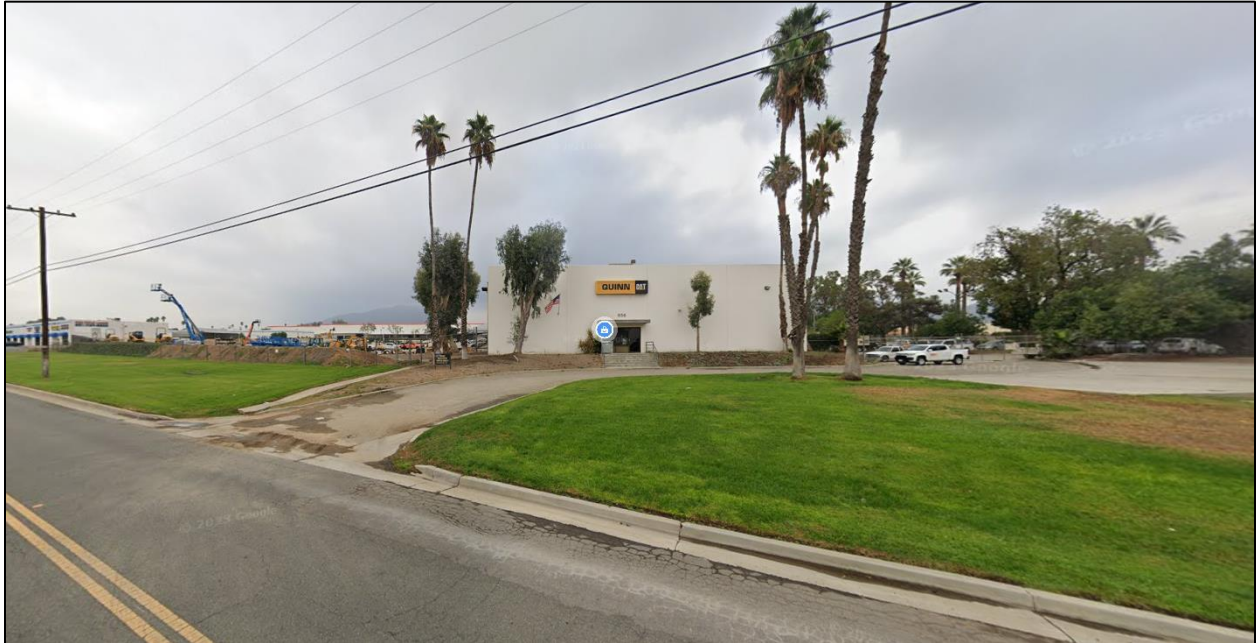
View from La Cadena looking at entrance of building (Quinn Power Systems)
