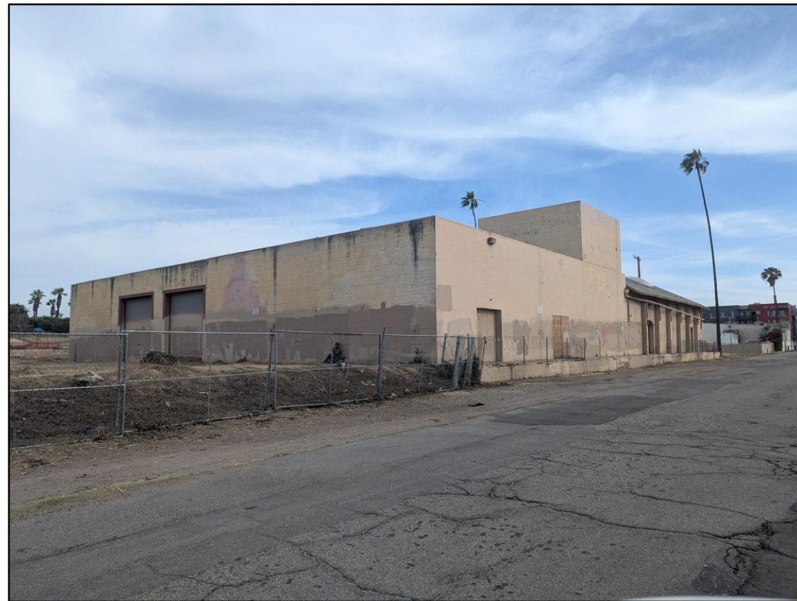
Non-original addition, looking southeast
