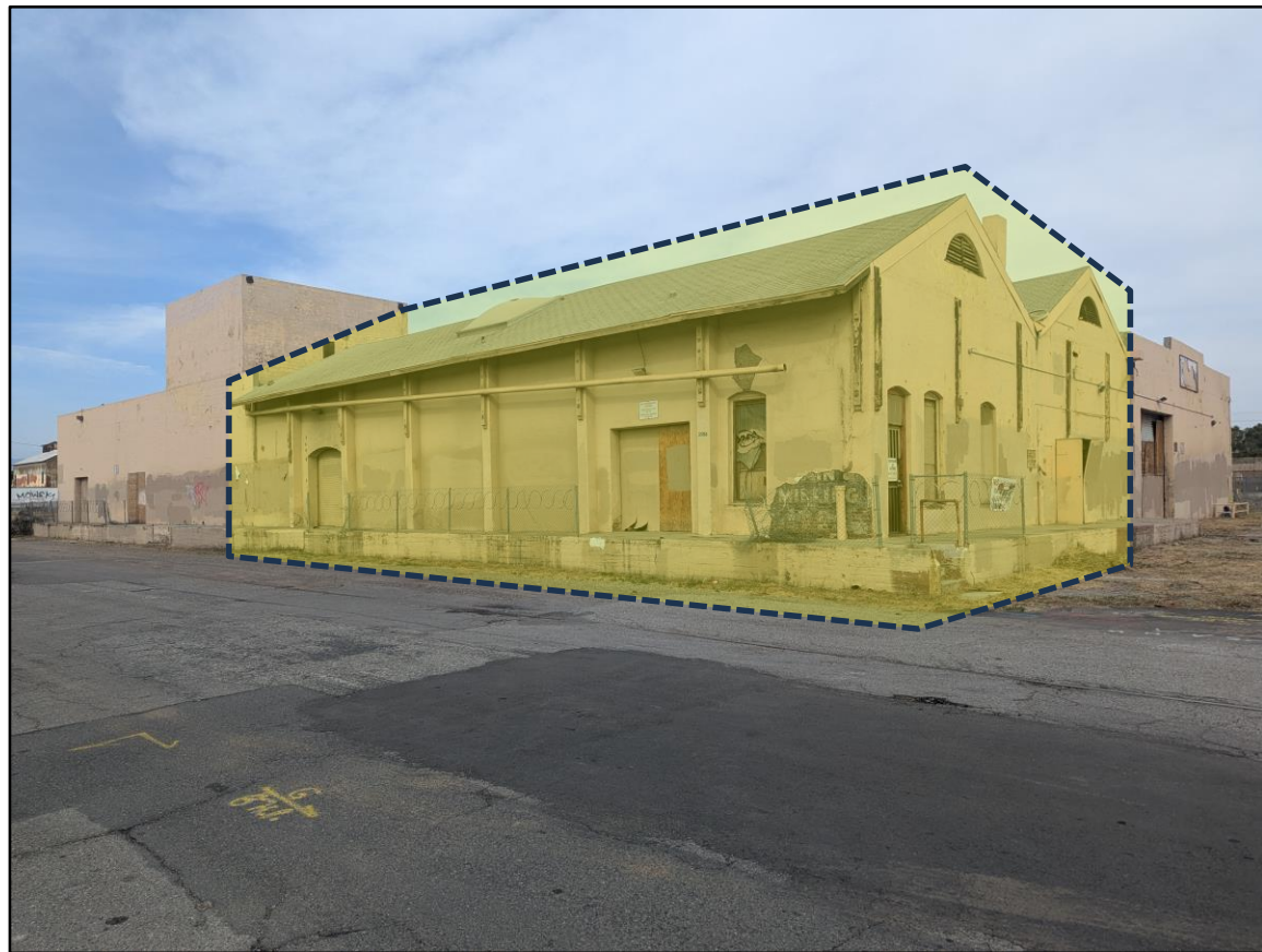
West and South Elevation, looking northeast
