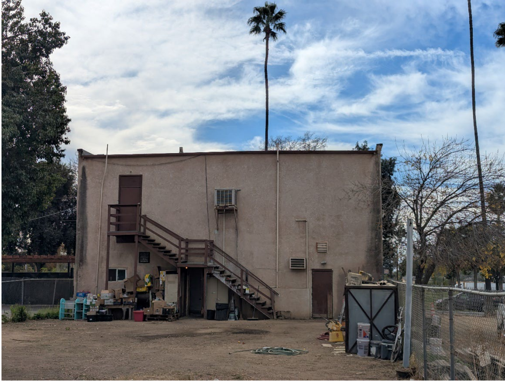
Figure 3 - Rear (North) Elevation, view looking south
