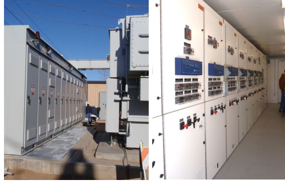
Proposed new transformer and switchgear
