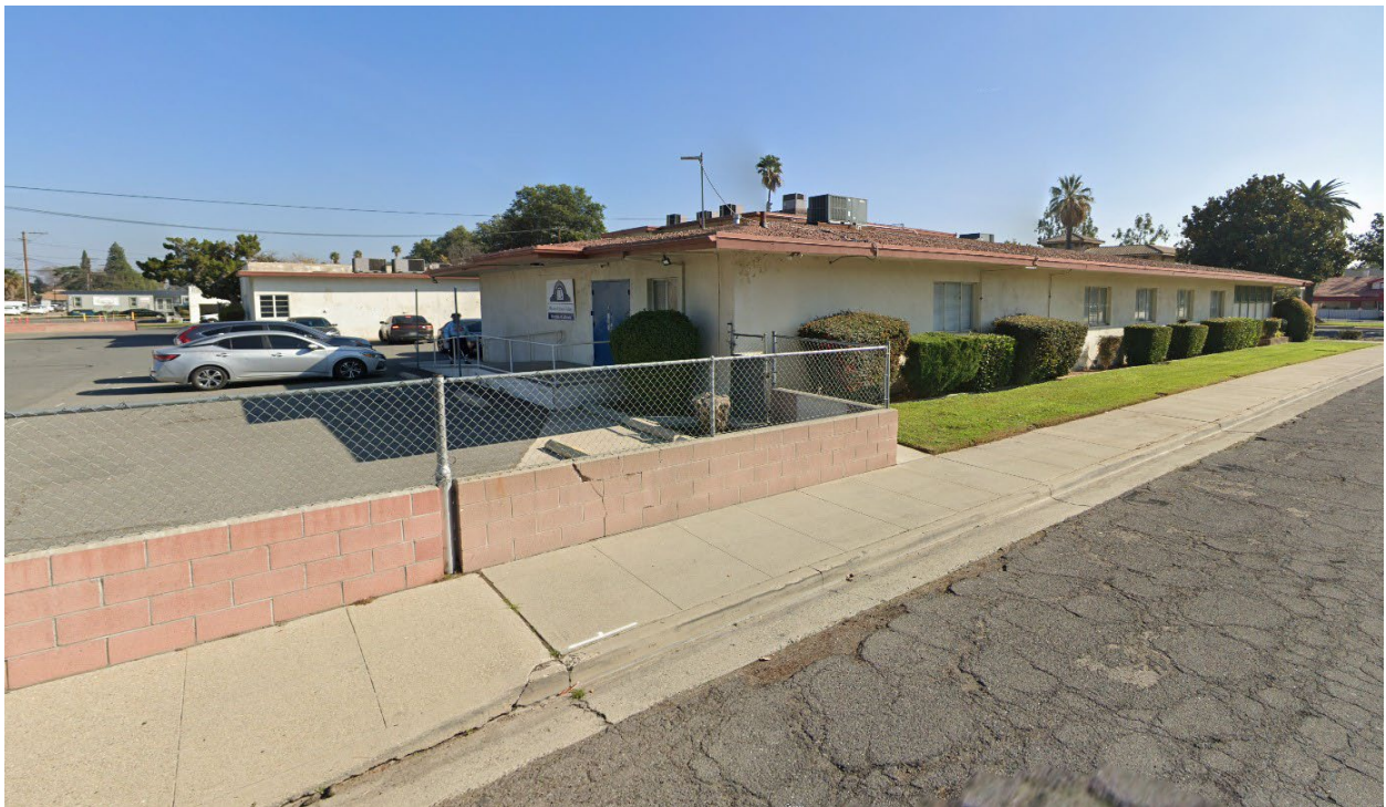
View of the project site looking northeast on Dykes Lane
