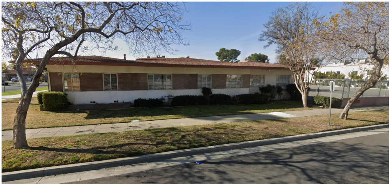
View of the project site looking west on Myers Street
