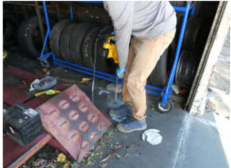
Photo #5: Rotomhammer drill installation of SS2 (southwest corner of tire shop)
