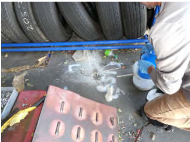
Photo #6: SS2 installation (southwest corner of tire shop)
