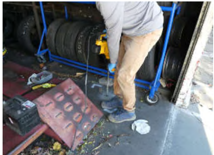
Photo #5: Rotohammer drill installation of SS2 (southwest corner of tire shop)
