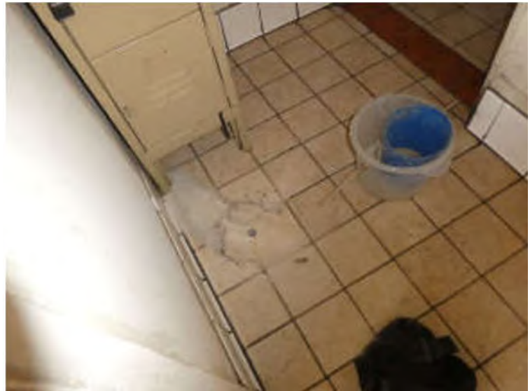
Photo #11: SS4 – Storage area of pizzeria
