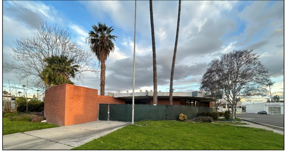
VIEW FACING NORTH FROM CENTRAL AVENUE
