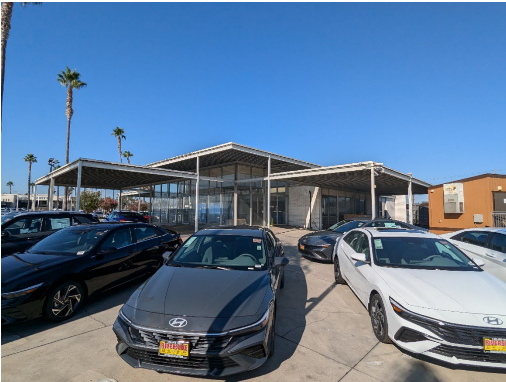
Figure 6 - East and North Elevation, view looking west
