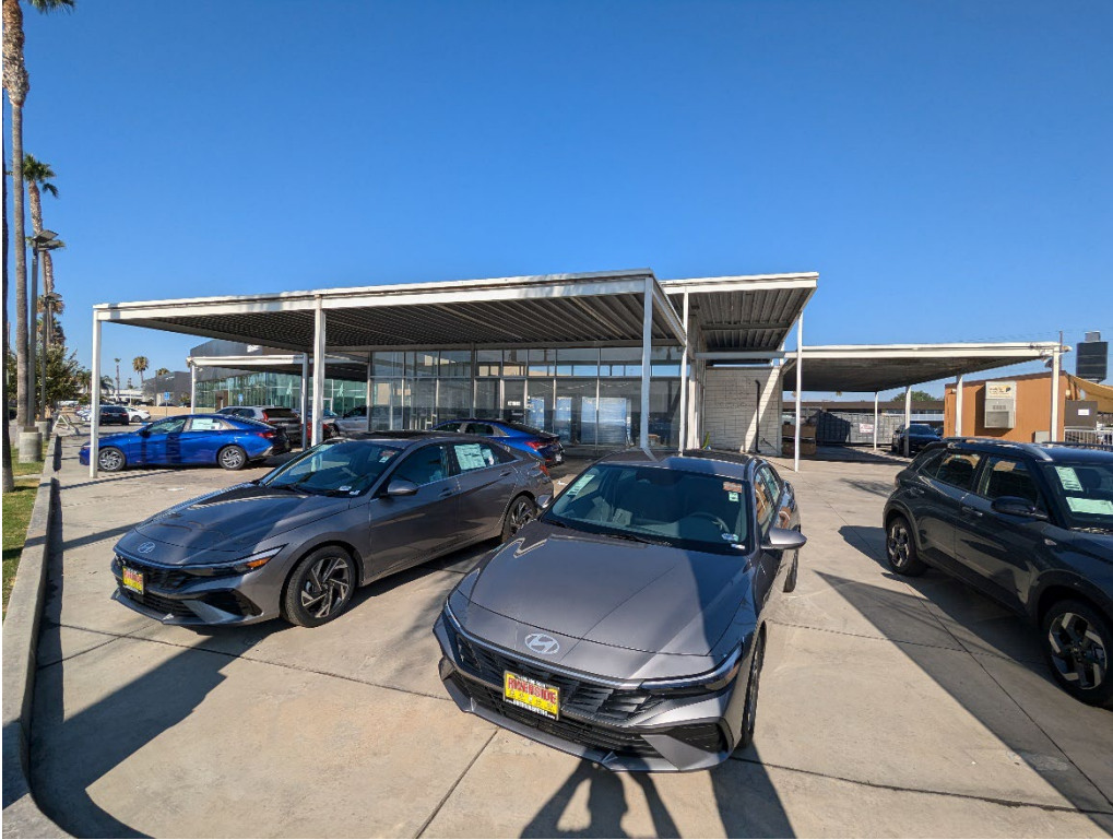
Figure 5 - East elevation, view looking west
