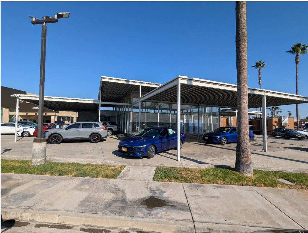
Figure 4 - East elevation, view looking northwest
