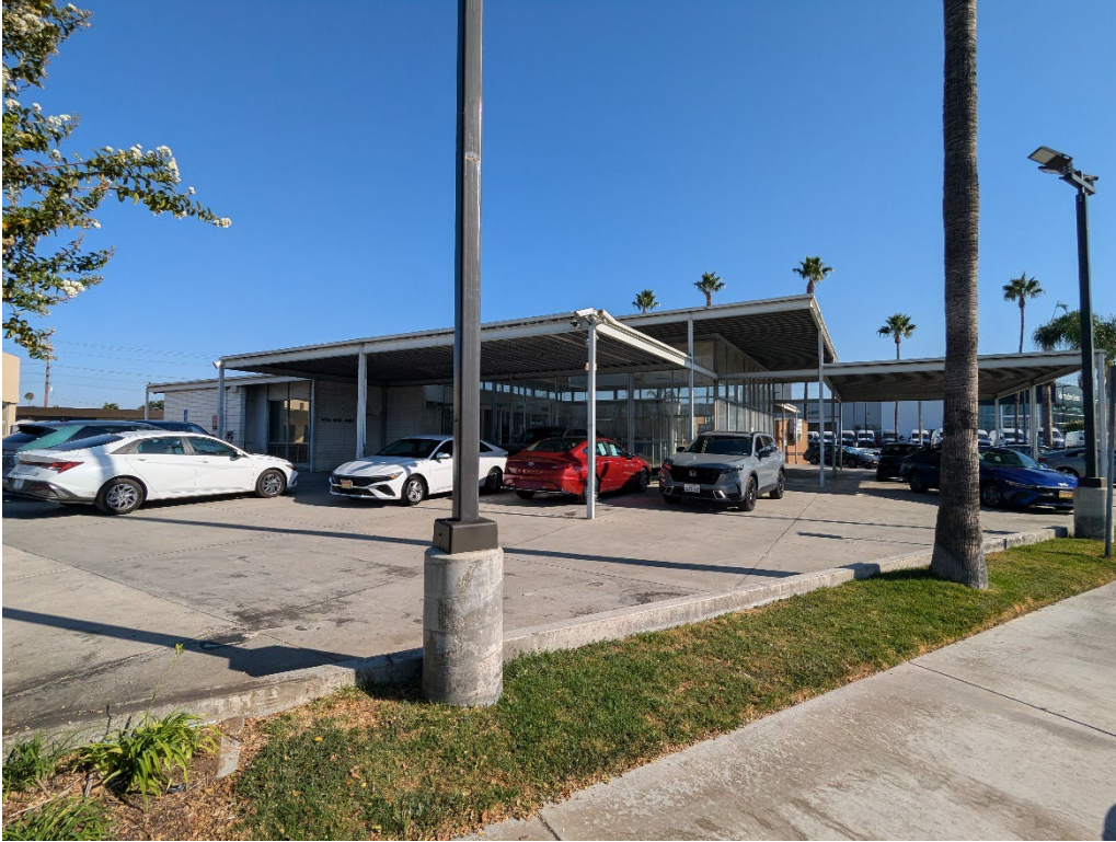
Figure 3 - South and east elevation, view looking north
