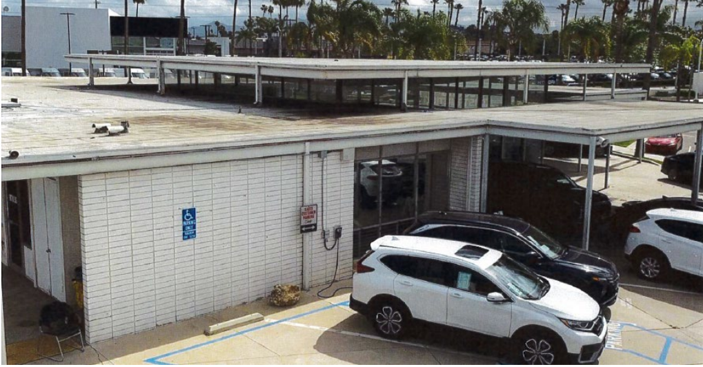
Figure 1 - Elevated view of south elevation, looking east
