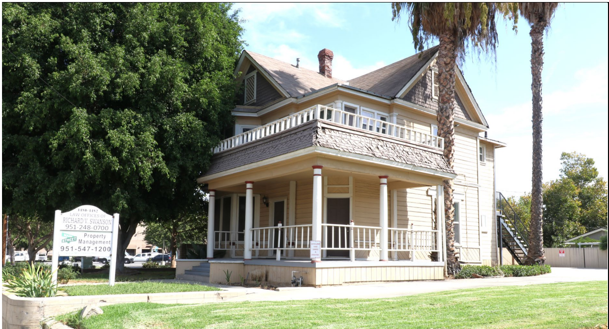
Photo 13. Offices at 4480-4482 Main Street, view northeast (10/7/24).
