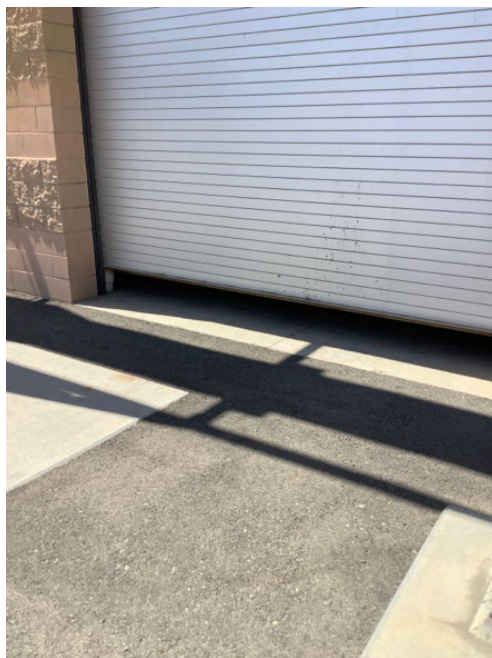
Photo 19: Layer 3 - Doors to some critical areas are left open to provide ventilation. This is a vulnerability, and there is a reliance on human interaction to ensure they are locked after hours.
