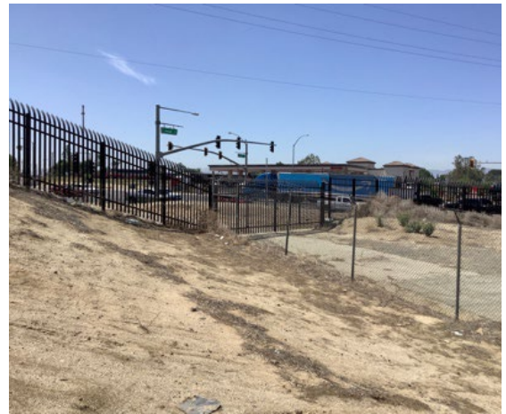
Photo 8: Layer 1 - The main fence is effective and meets best practices. The secondary fence shown here is unnecessary.
