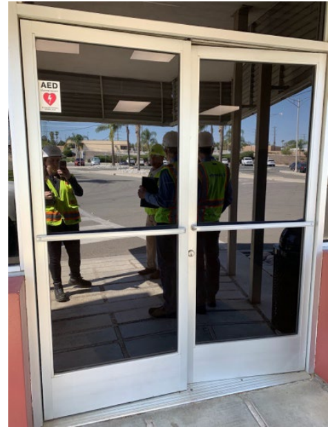
Photo 22: Layer 3 - Windows and doors with windows are too easily circumvented.
