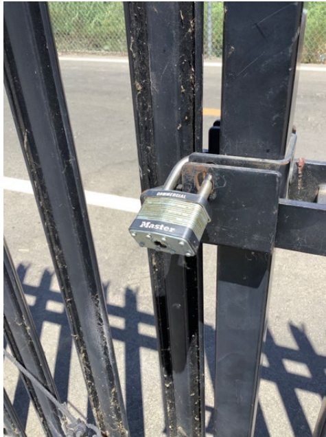
Photo 9: Layer 1 - Padlocks on man gates are not very strong and can be cut.
