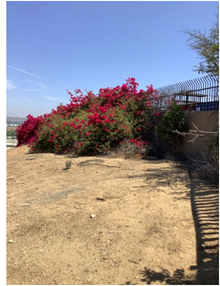
Photo 6: Layer 1 - CPTED concerns with vegetation on perimeter. Allows entry, hiding spots, and inhibits surveillance.
