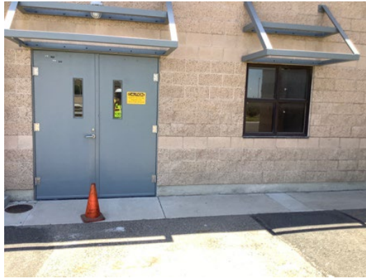
Photo 21: Layer 3 - These doors are an example of strong physical security for entry points. They are metal, in metal frames, and have a full astragal.
