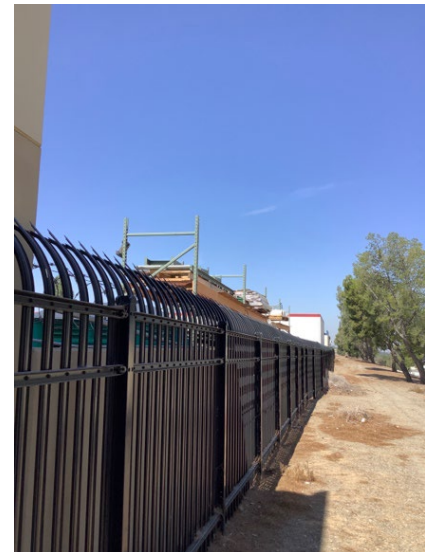
Photo 4: Layer 1 - Fence is defeated by equipment piled outside it.
