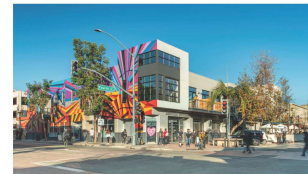
4TH STREET MARKET LOFTS LOOKS BEACH (RETERIOR)
