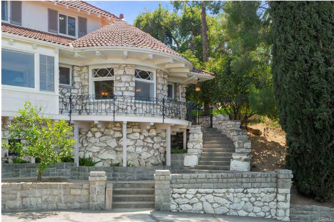
Figure 11 - Rear elevation steps, view looking southeast
