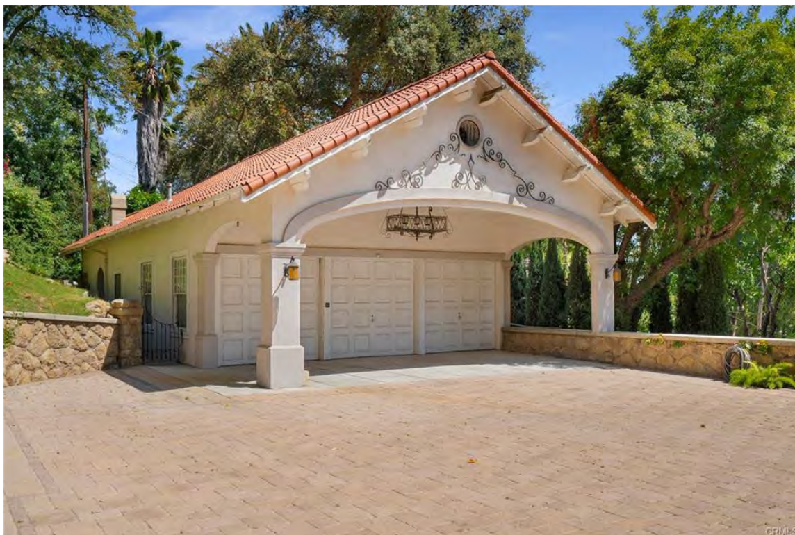
Figure 19 - Garage, view looking west
