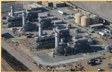
Riverside Energy Resource Center (RERC)
