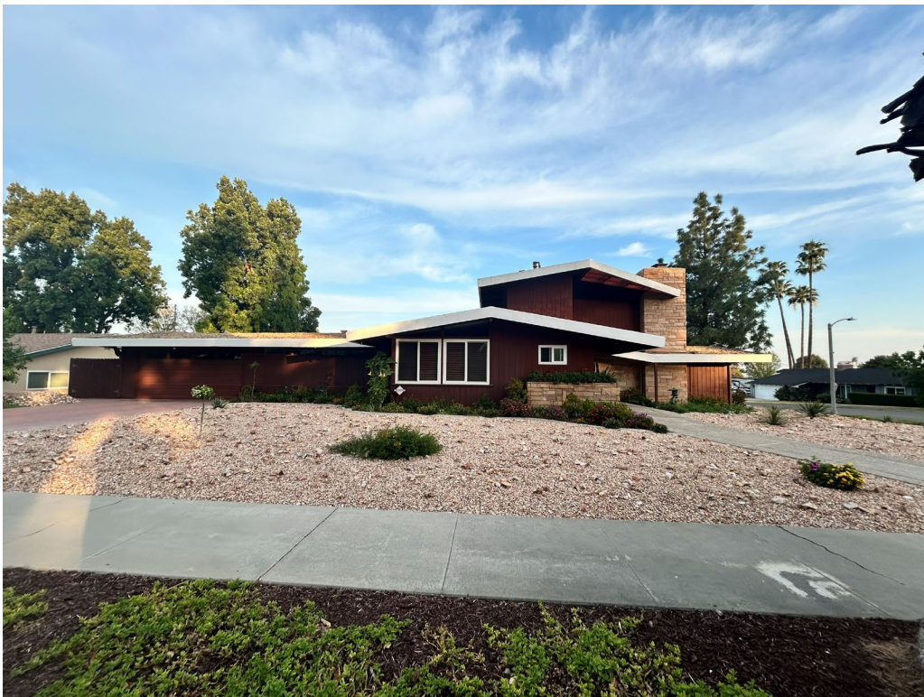
Figure 2 - Primary (south) facade, view looking northwest
