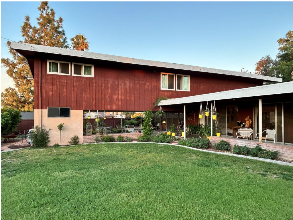
Figure 6 - West elevation, view looking northeast
