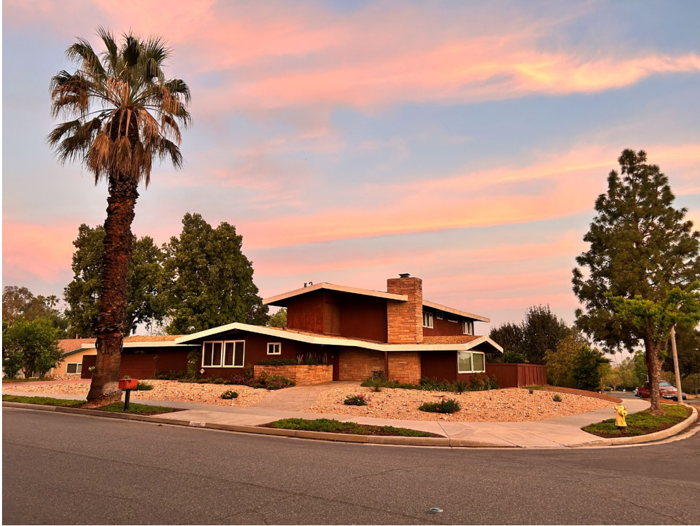
Figure 1 - Primary (south) and Secondary (east) facades, view looking west
