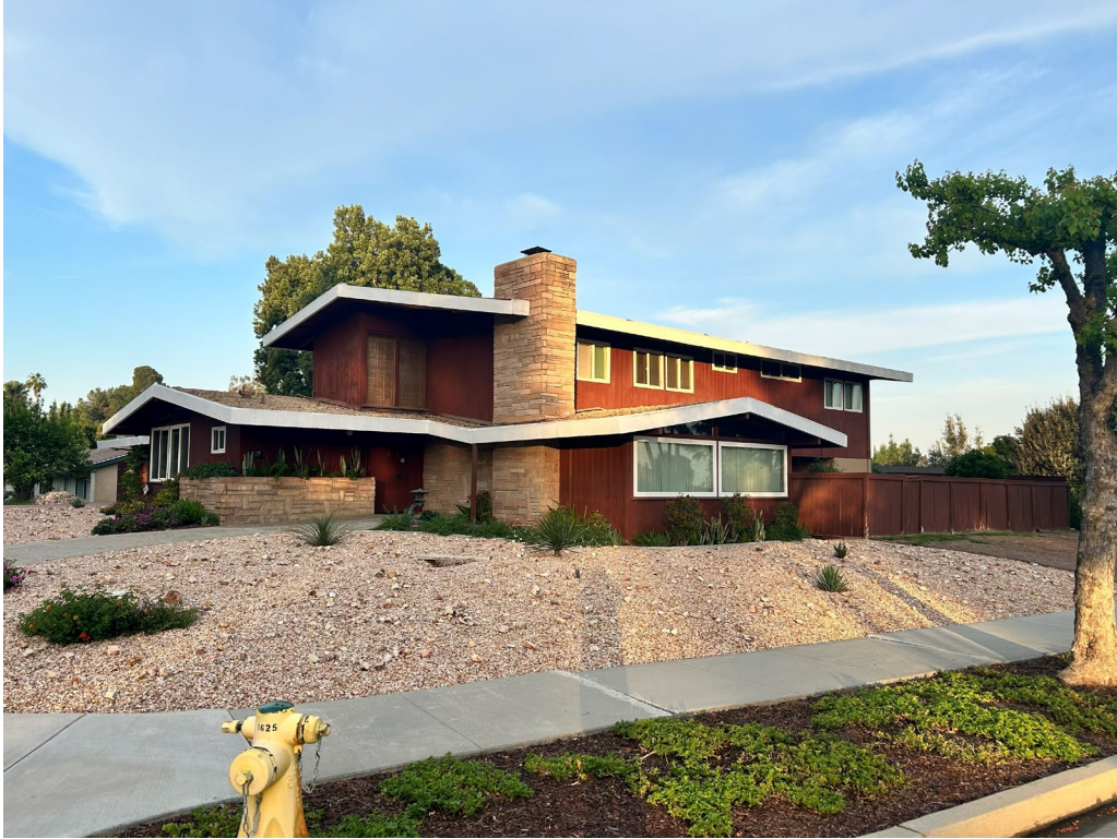
Figure 3 - Secondary (east) facade, view looking west
