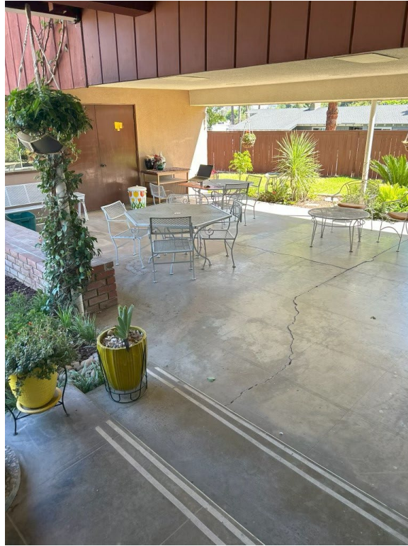
Figure 9 - Patio under second story
