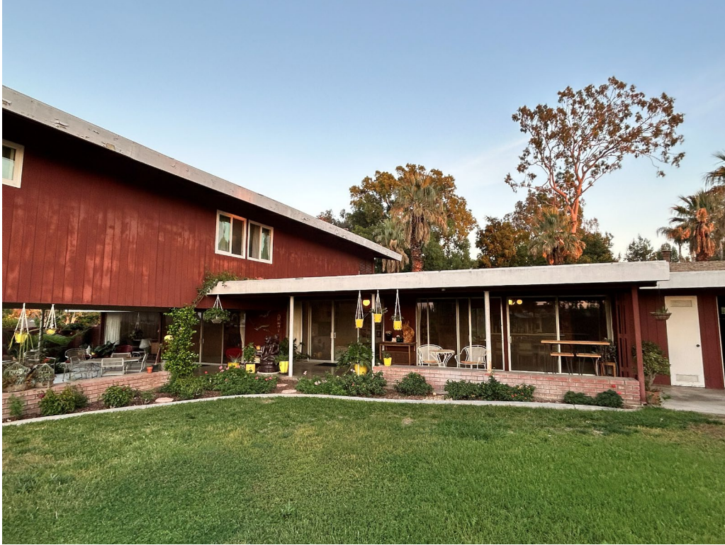
Figure 7 - North elevation, view looking south
