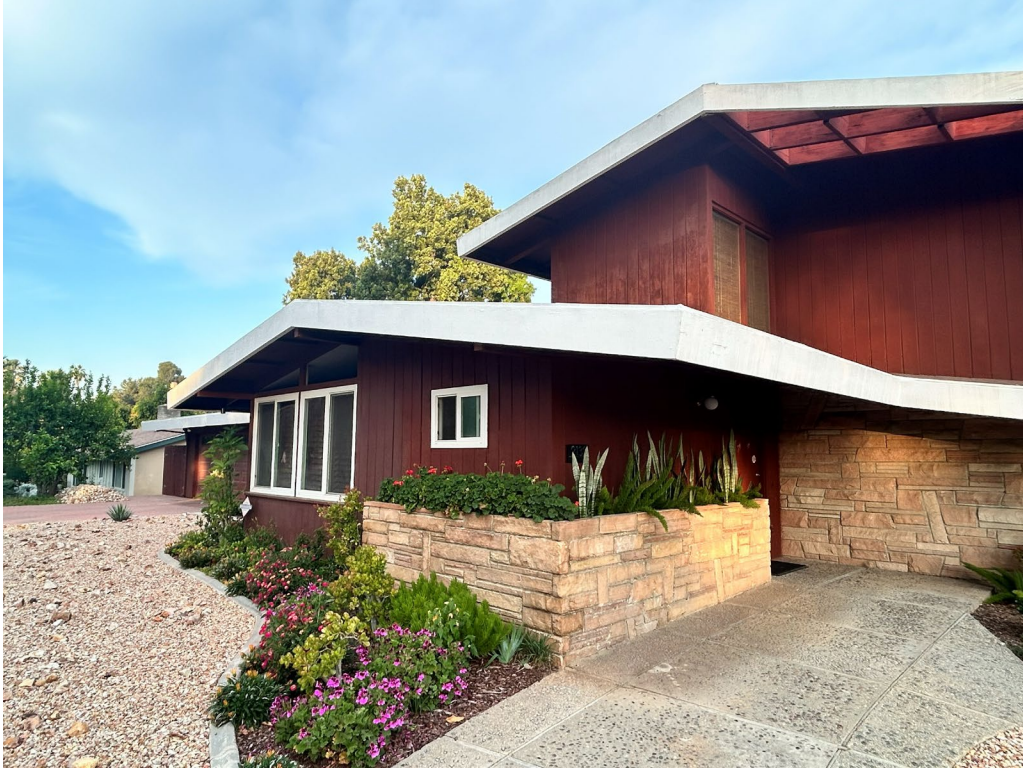
Figure 5 - Main entry, view looking west
