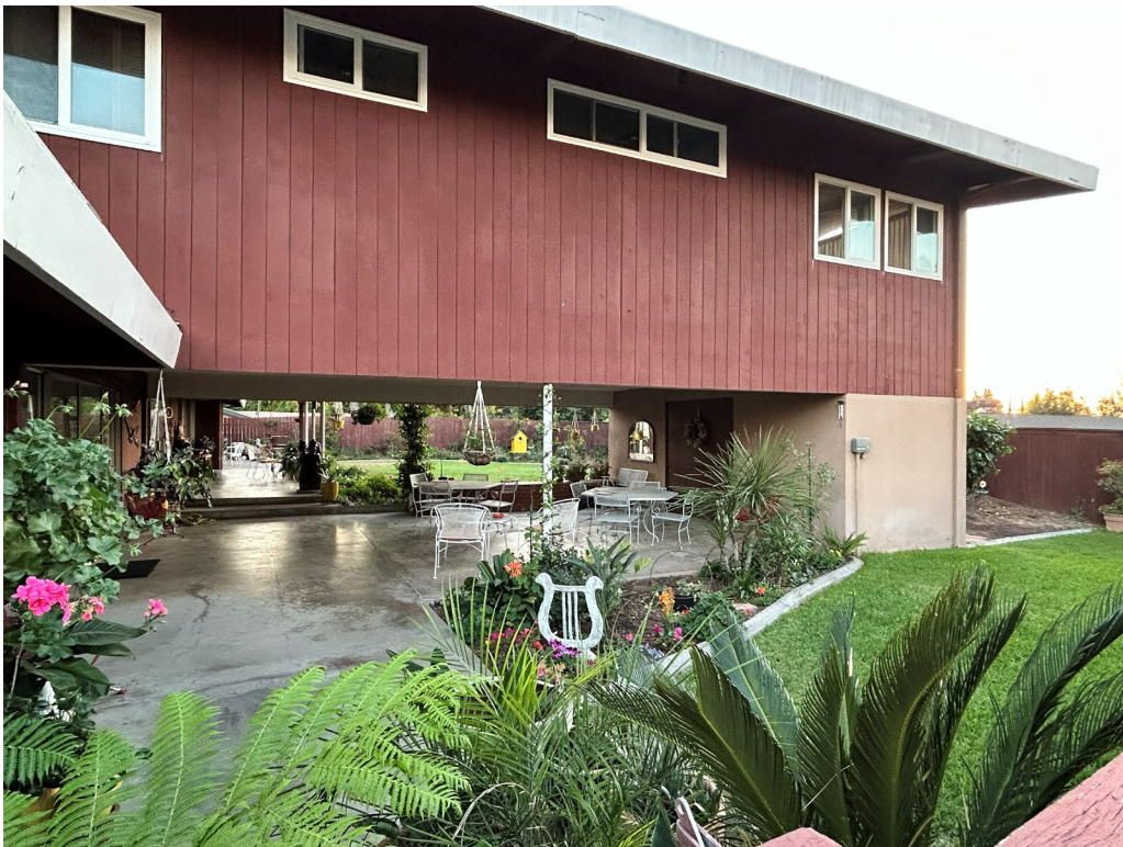
Figure 8 - East elevation, view looking west
