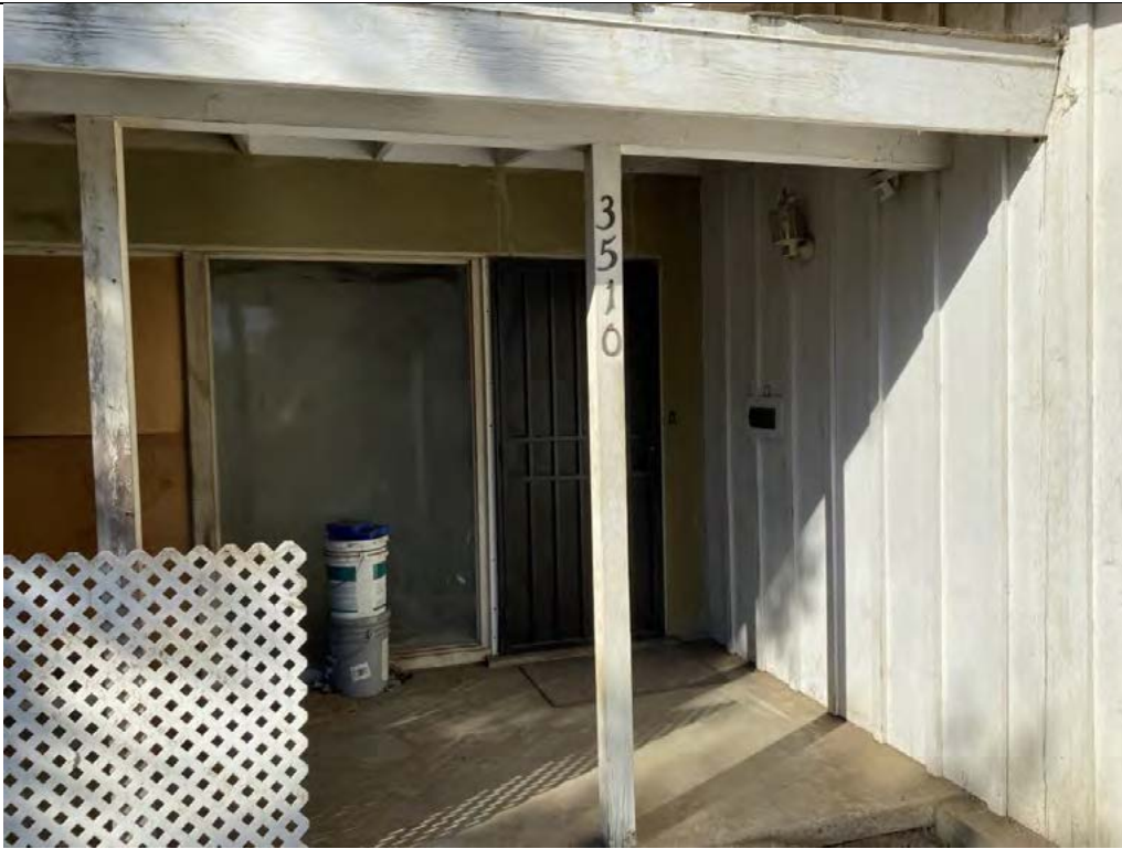
Photo 22: View of northern property structure closeup facing west.
